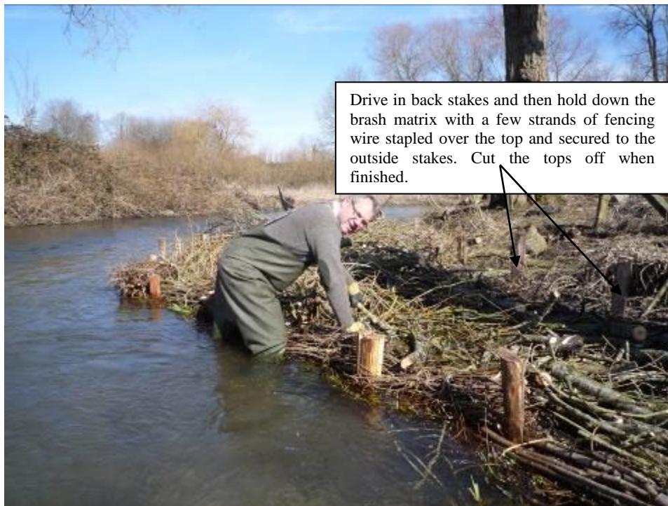
Photo 12 Packing a marginal shelf with lots of wood brushings to help collect sediments and provide a medium for marginal emergent plant growth.
