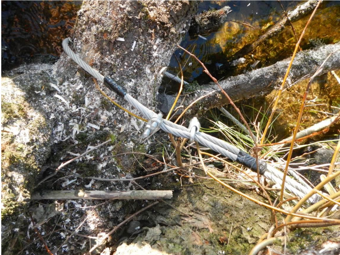
Photograph 22. Stump cabling for a tree kicker.
