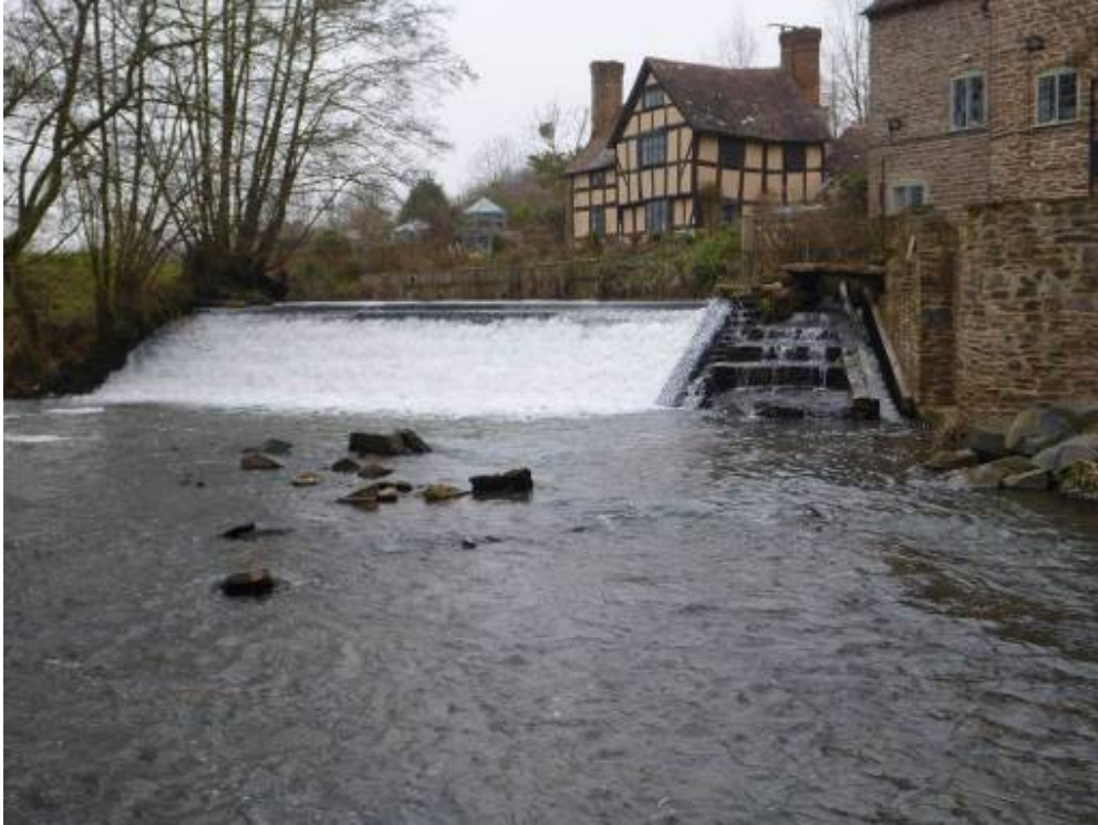
Photo 10 Detton Mill weir with an Alaskan fish pass (right of picture) and eel pass (right of white water). There was very little attraction flow from the fish pass at the time of the visit.
