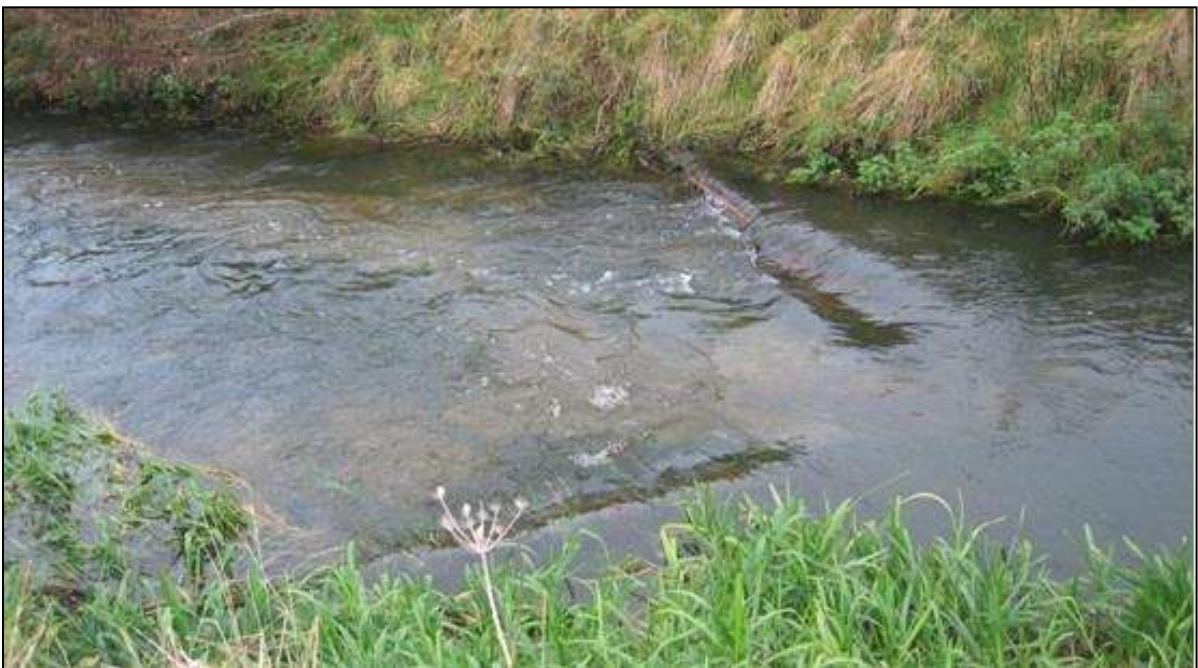
Figure 19: An example of a pair of deflectors in an upstream-facing V formation
