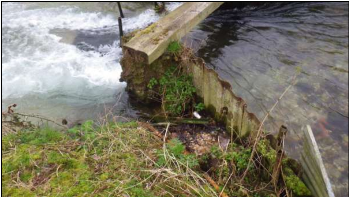
Figure 4: The weir is in poor condition and the river is cutting around the sides
