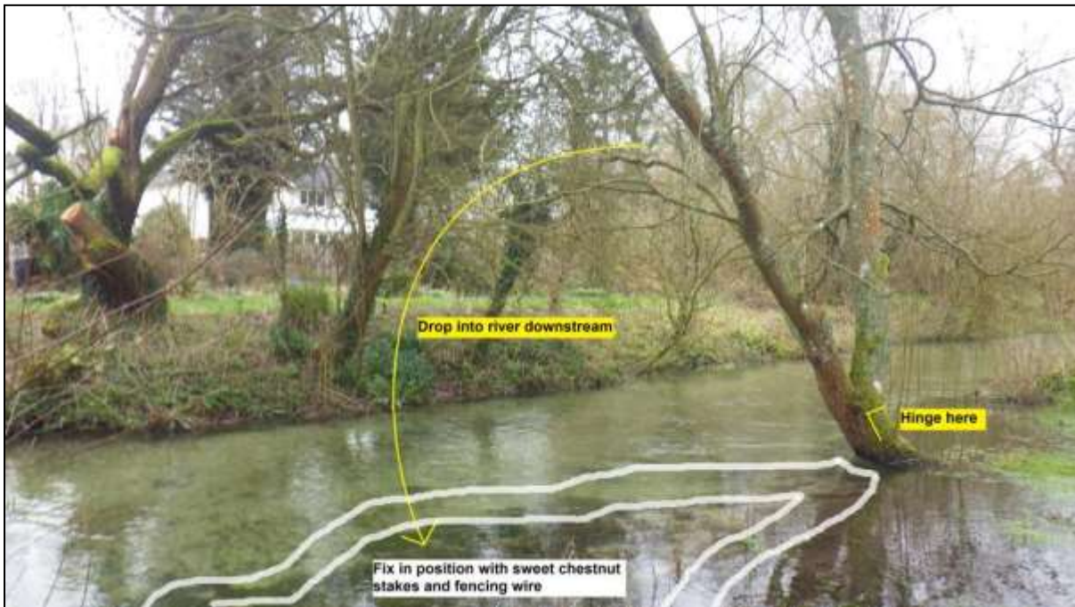
Figure 15: An example of an existing tree that could be hinged into the river.
