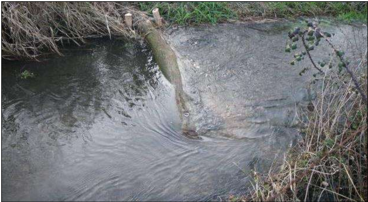
Figure 16: An example of a simple log deflector. Note the bankside edge is keyed into the bank and the log slopes down into the river. The stream flows from left to right in this picture.
