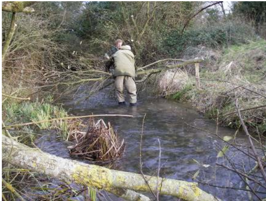
Installing brushings designed to provide improved cover for spawning trout and their offspring on a tributary of the Wylfe. This could be a way of providing temporary cover until thicker marginal cover has established.
