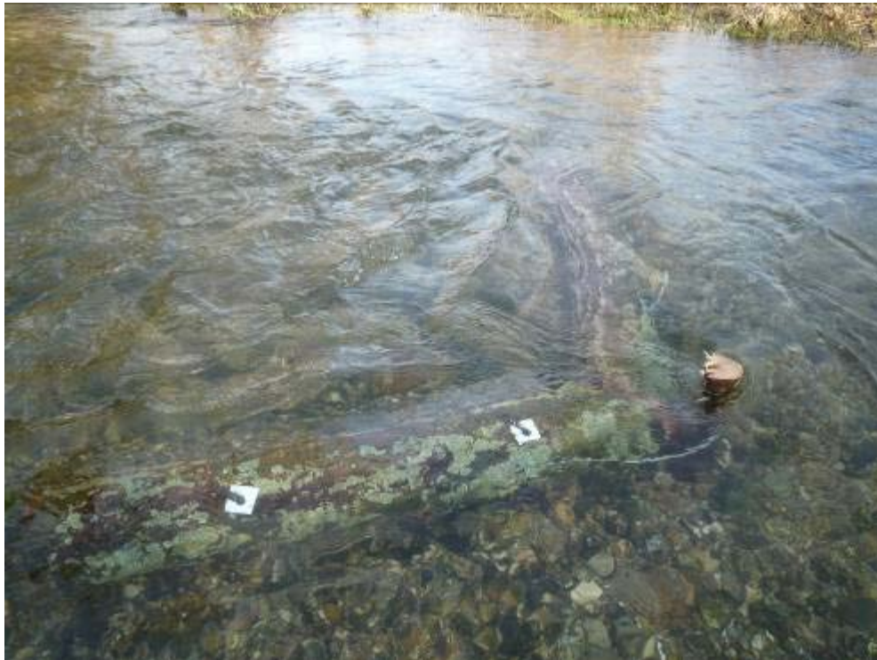
Two pieces of LWD configured to form an upstream "V". Structures like this scour local pots in the shallow bed and promote a clean, loose ramp of gravel downstream.
