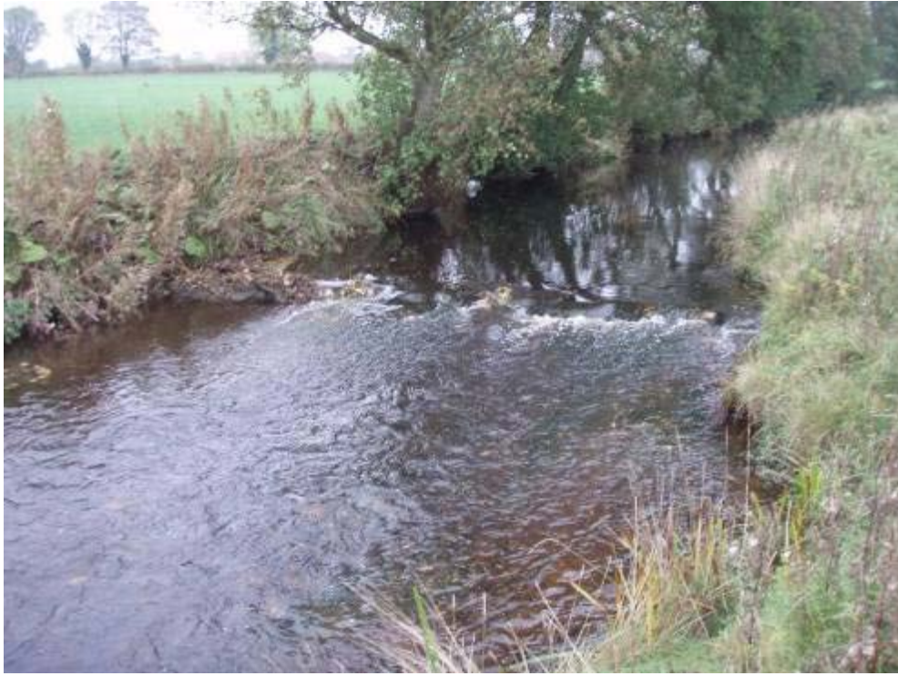
Photo 4 Low stone weir on upper river section. Replacing such structures with groynes would reduce water impoundment and improve in stream habitats.
