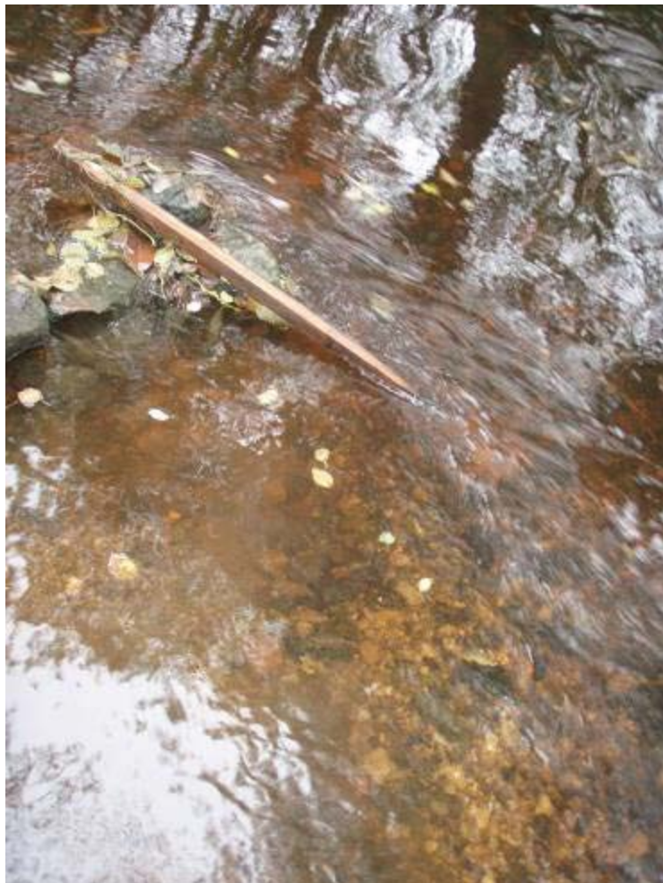
Photo 11 Stub groyne can clean and sort gravel and improve spawning success
