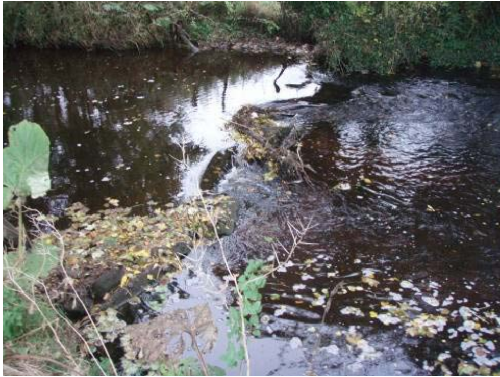
Photo 12 Low stone weir in the fishing hut field – replacement with a series of log groynes would reduce impoundment and provide a more varied habitat
