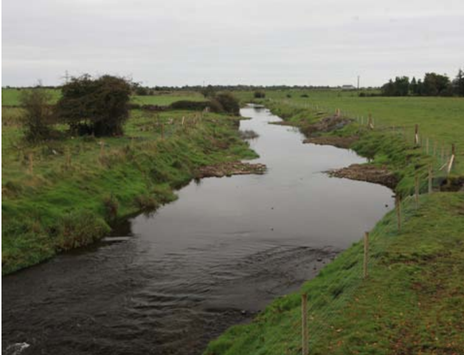
Boulder deflector ‘pinch points’ with rubble mats installed by IFI on the River Robe
