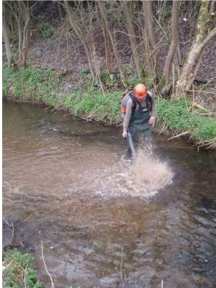
Cleaning spawning gravel using a mechanical leaf blower.....
