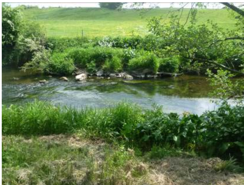
Figure 4 Effective use of boulder and gravel to constrain flow and create scour without upstream impoundment
