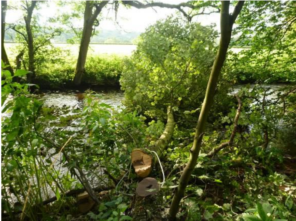
Photo 3. A large sycamore deliberately dropped into a Welsh spate river and cabled to its own stump.
