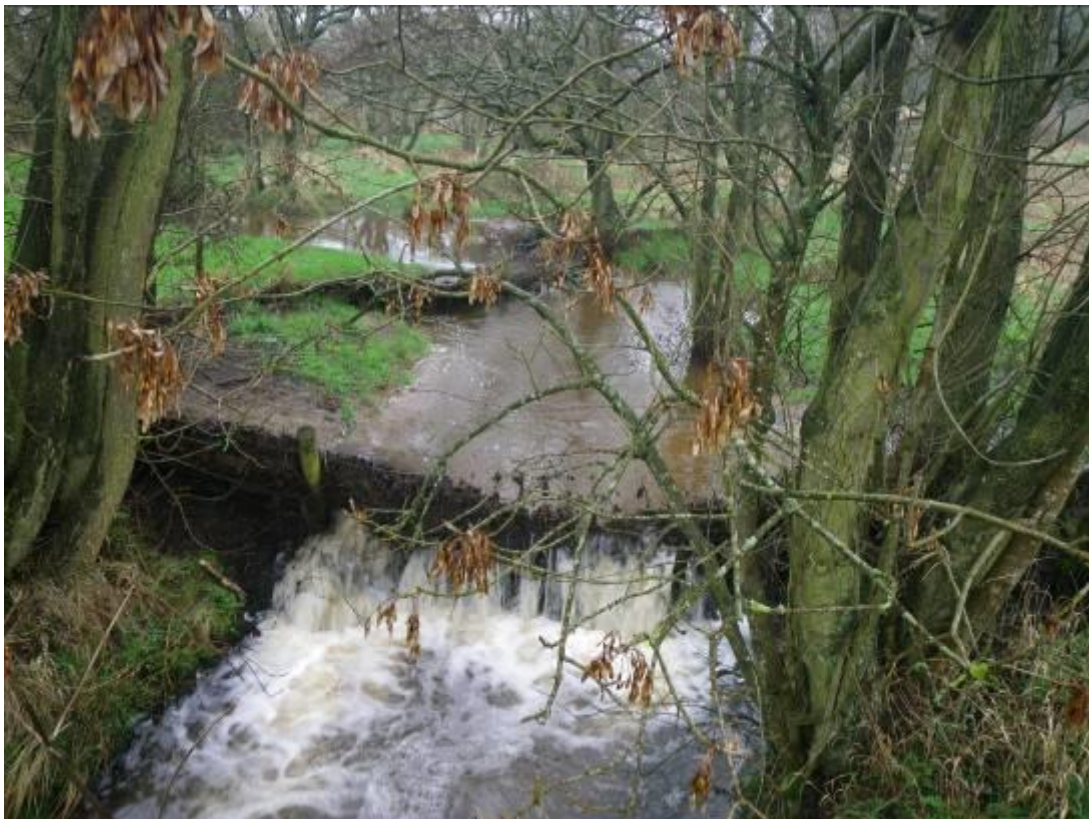
Photo 6. A sheep fence causing a debris dam to form, creating problems for fish migration and also resulting in the river bed levels rising upstream.
