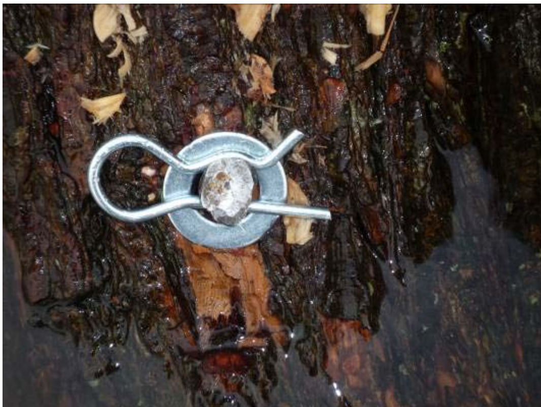
Cross drilled and pin method
