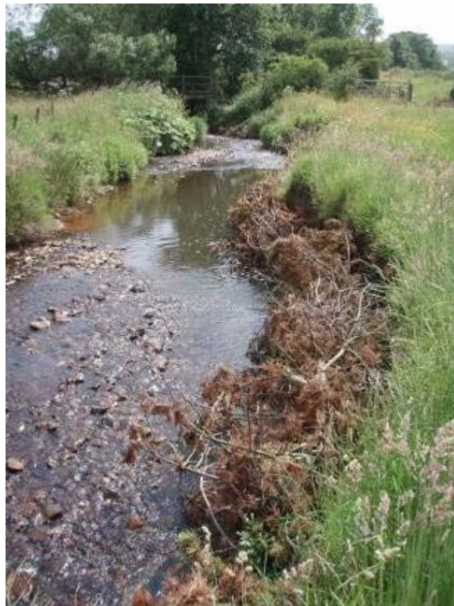
A large eroded bend on the Monnow at Pandy defended with “whole” tree revetment
