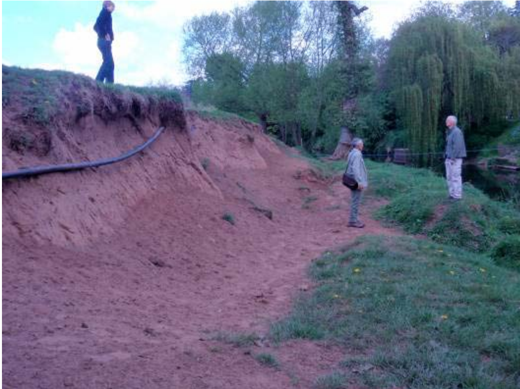
Eroded bank with exposed water pipe. Note the river bank margin appears to be relatively stable at this location.
