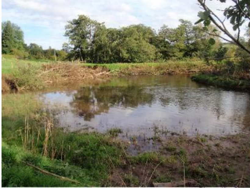
A large eroded bend on the Monnow at Pandy defended with “whole” tree revetment
