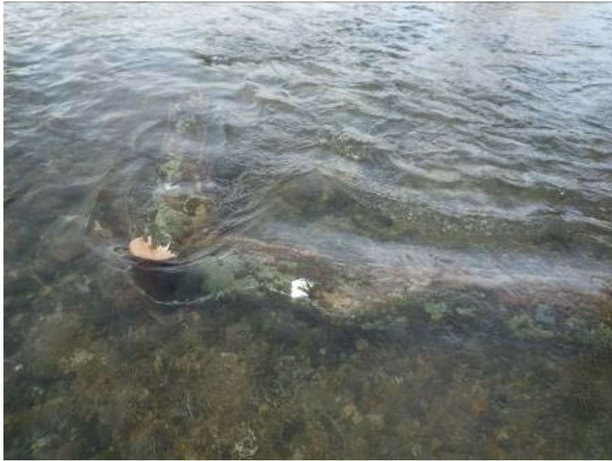
A short upstream facing "V" structure pegged onto a gravel run and designed to improve spawning opportunities. These structures also create small holding pots for spawning adults and holding lies for juvenile trout
