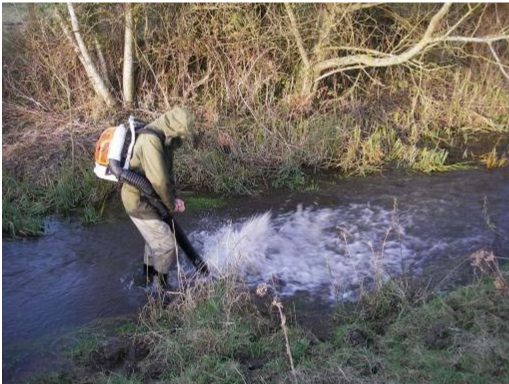
Gravel cleaning using a back pack leaf blower. Cleaning gravels on the top beat is recommended
