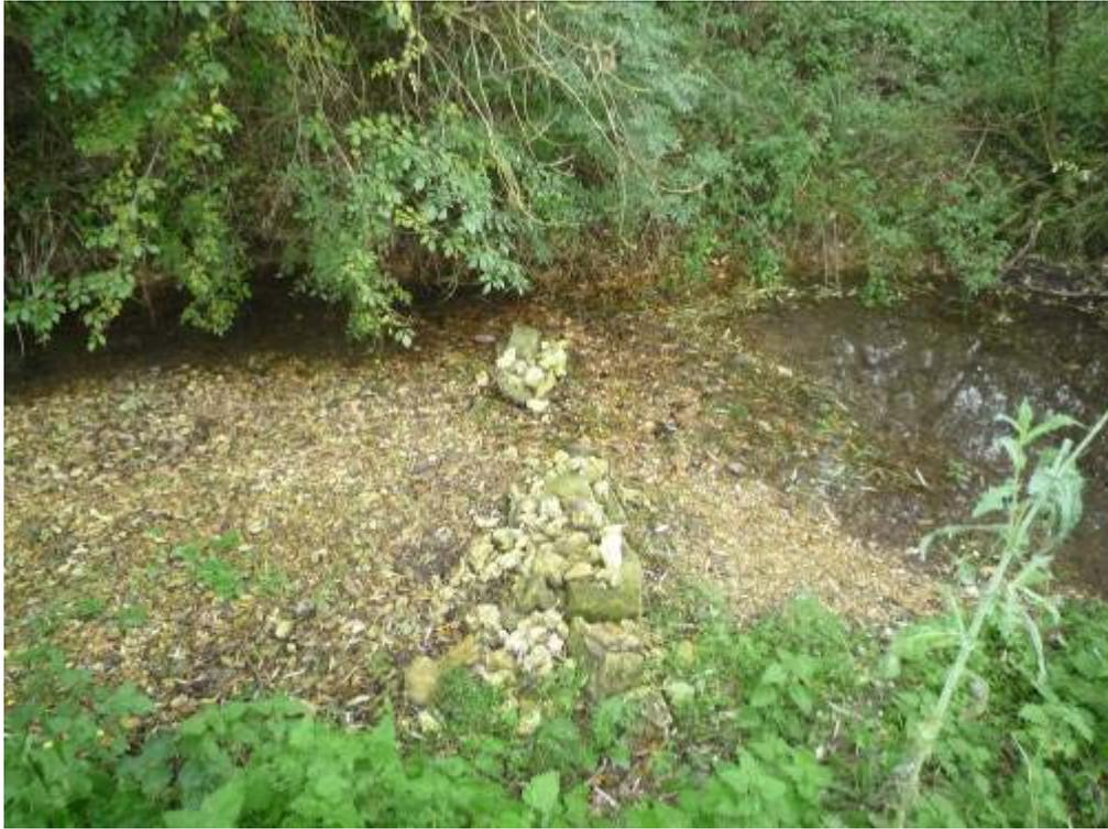
Pic 1. A section of dry channel where some stone groynes have been installed by the previous owner in an attempt to locally increase water velocities.
