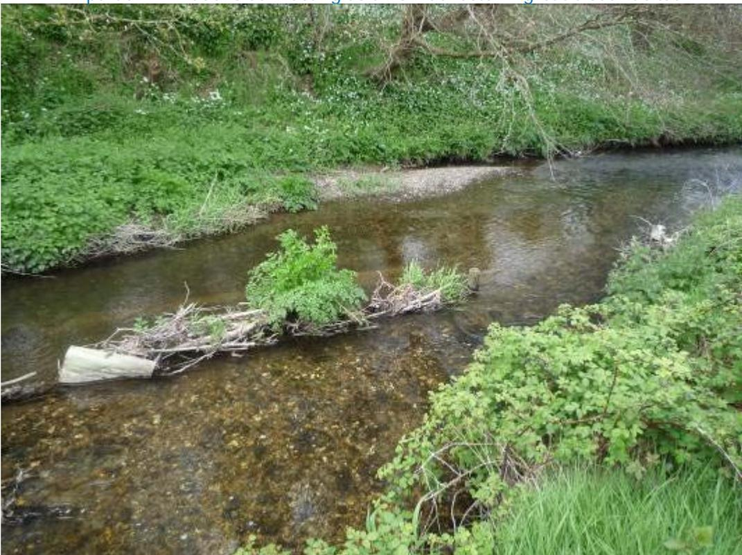
The remains of some old inchannel flow deflectors. These are much more effective when placed at right angles to the flow or pointing slightly upstream.
