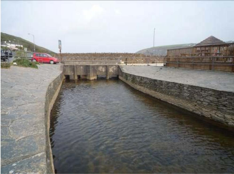
Downstream view of the same structure – Note the limited flood capacity caused by the restricted flow through the small apertures
