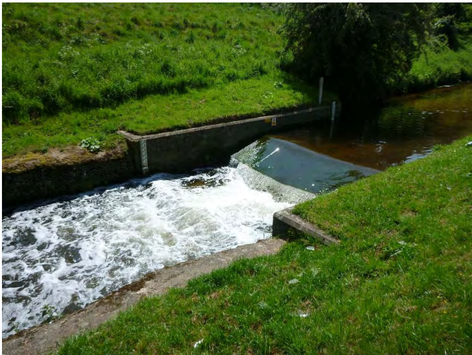
Photo 10 Flow gauging weir at SK5587763487. This is a barrier to fish migration. If the weir face was continued down to the bed, a low-cost baffle array could be fitted, or the weir replaced with an open-channel flow gauge.
