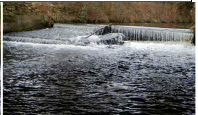
Photo 4 Ollerton Road Bridge 1
