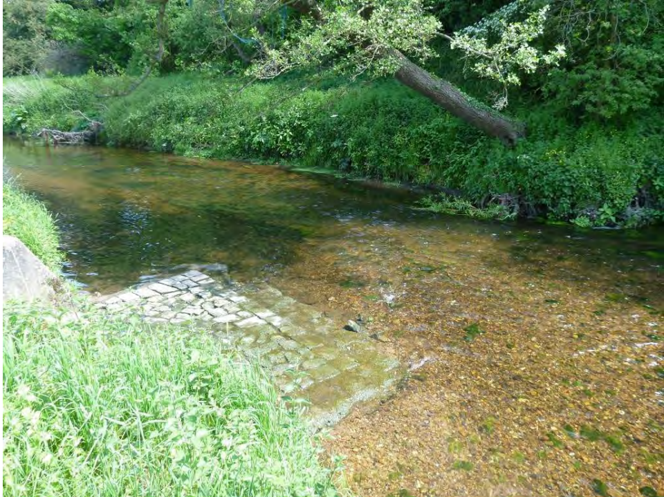
Photo 9 Pinch points in the channel, such as this spillway beneath an outfall, create increased scour and depth, providing better adult fish habitat. The bank stability and cover provided by the tree and roots on the far bank enhance the effect. Note how the width u/s allows the retention of gravels and potential spawning areas, while the pinch creates scour that creates and maintains pool depth.
