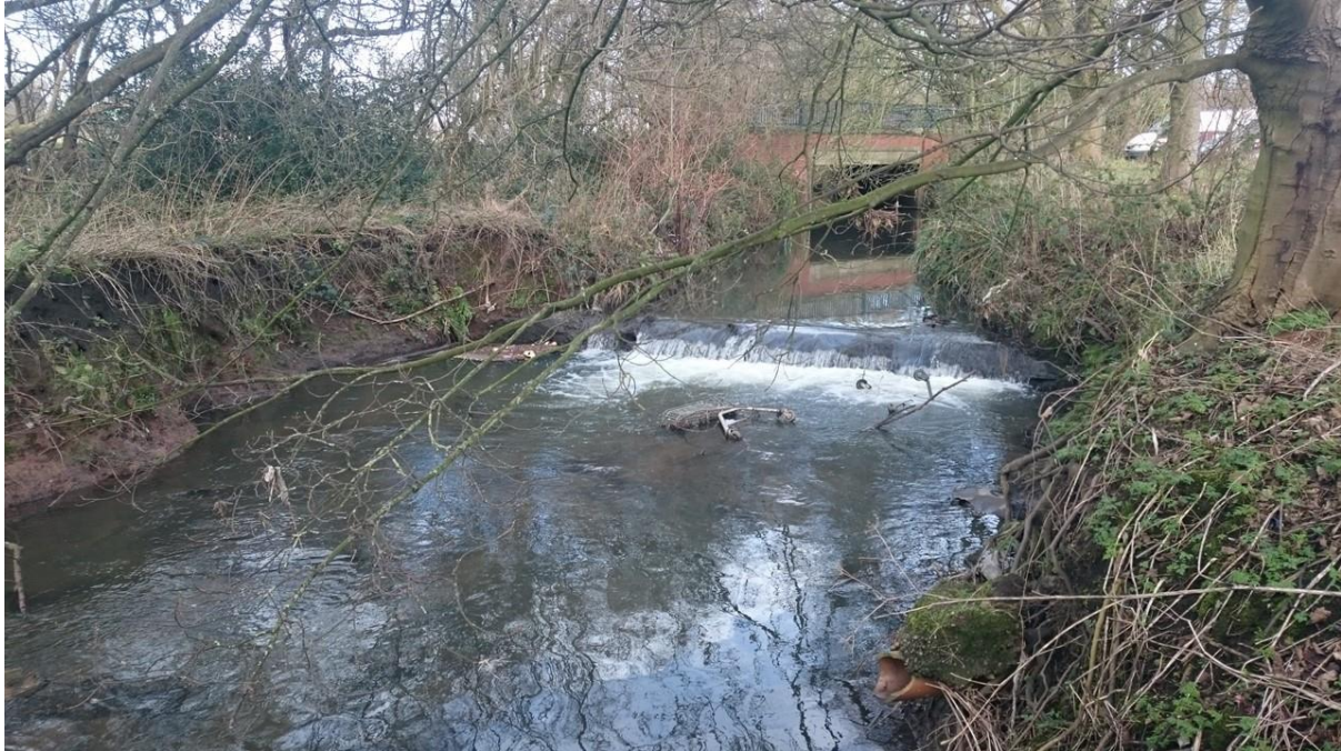
Figure 2: The white water (entrained air) below the weir combines with the height of the weir crest to make this a more significant barrier to migration than most observers appreciate. The impounding effect extends far upstream of the road-bridge (Clayton Lane) visible in the background. The erosion (particularly on the RB which is pictured on the LEFT of this photo) is caused by the construction of the weir at right-angles to the original river banks and the soft nature of those banks.
