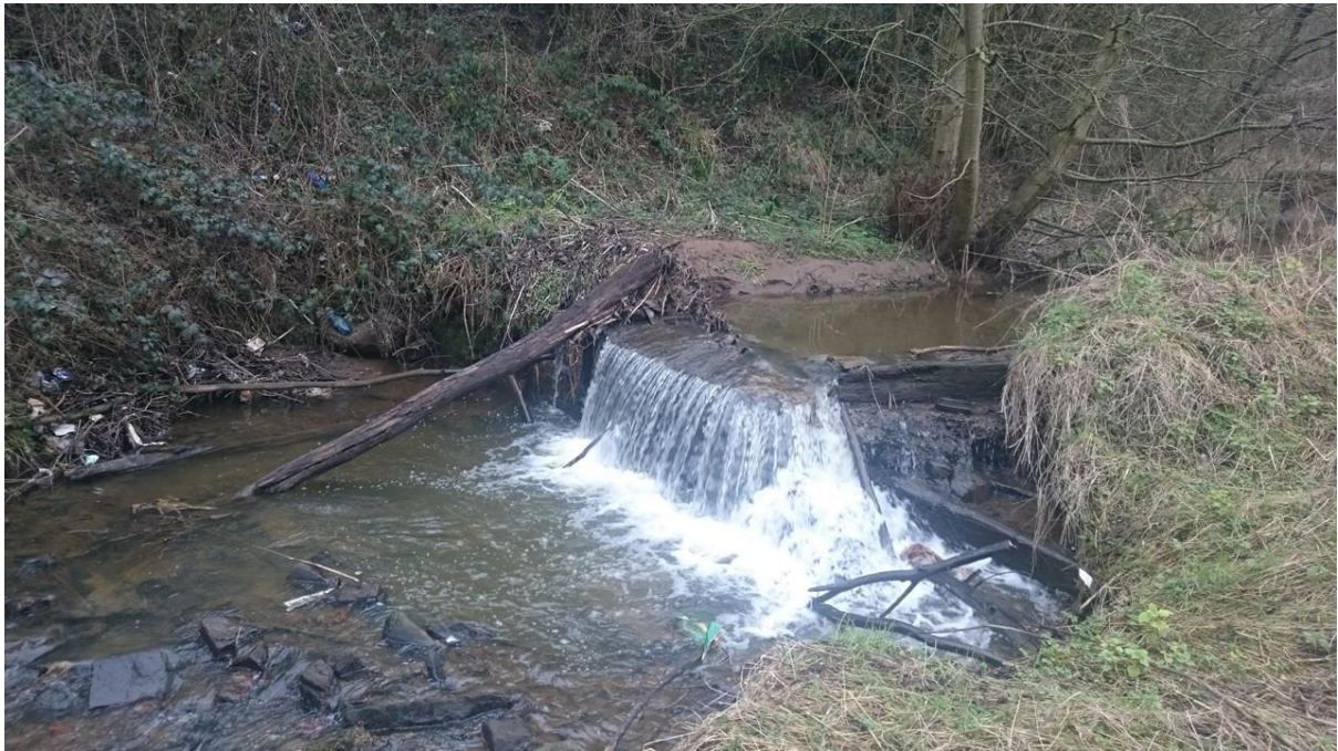
Figure 3: Causley Brook Weir 1 at SJ 85779 44170 – concrete and wood structure
