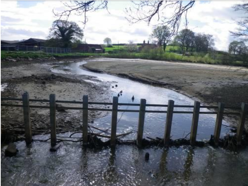
Photo 3 View of the drained down Mill Pond with huge quantities of settled sand. This area could be either a “green swale” or alternatively a small “off-line” pond but would still provide additional capacity during a large flood.
