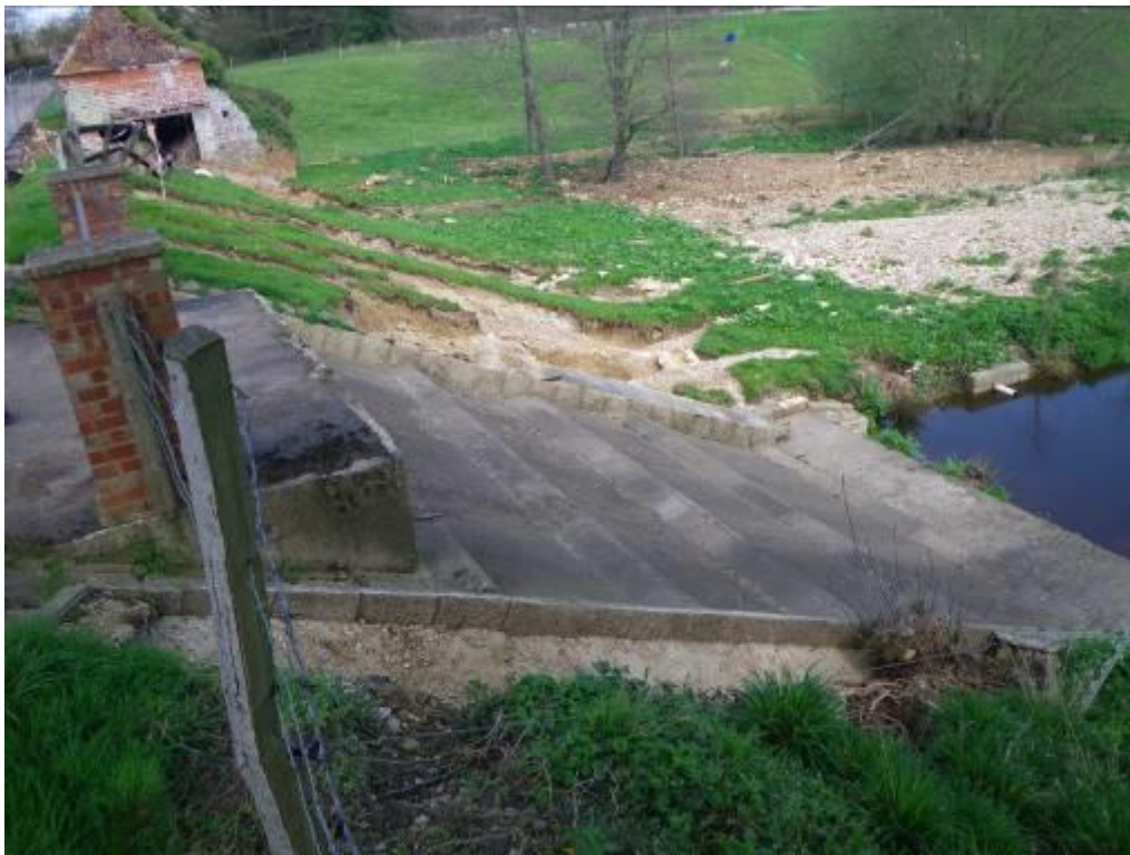
Photo 8 High level spillway outlet. This could be broken out to create the new route for a naturalistic river channel.
