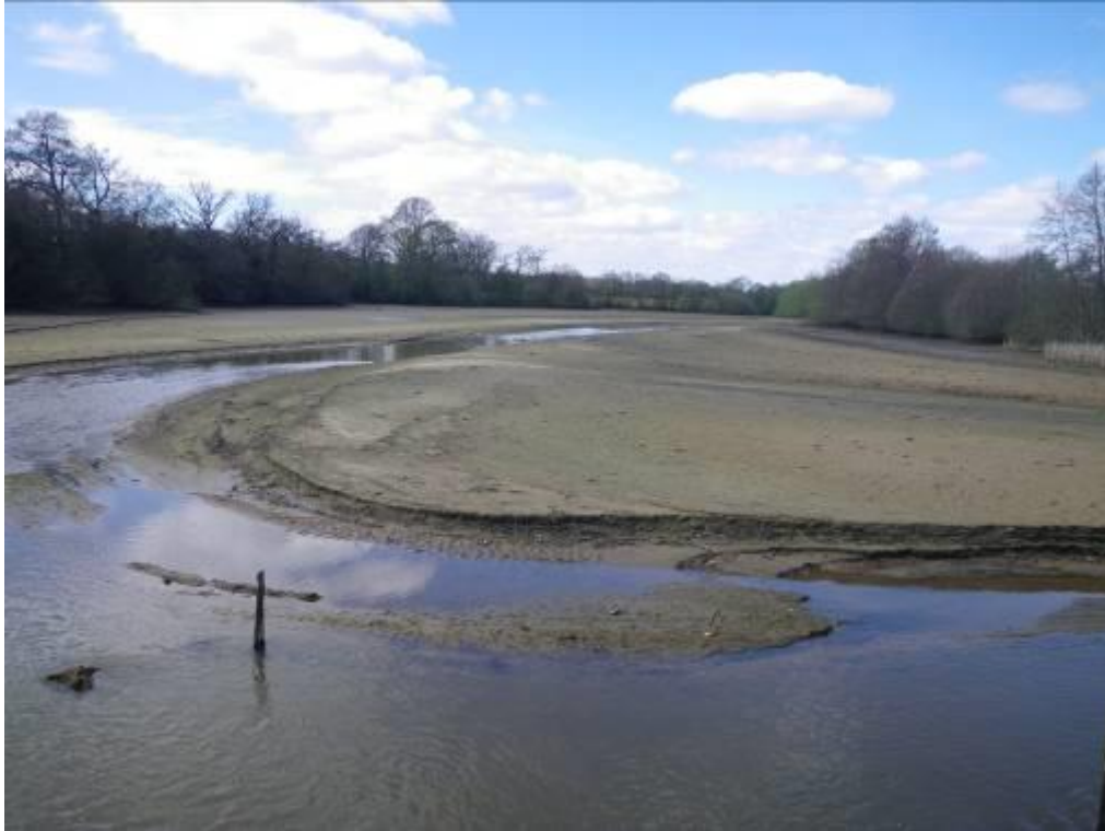
Photo 12. View upstream from the spillway. A new river channel with small managed “steps” in the bed to overcome the existing head differential could be created both downstream and within the bed of the old mill pond. Soft river margins would have to be defended with biodegradable geotextile and planted. The area to the right above could be raised to separate the channel from an excavated off-line pond if this is deemed an essential element of the project.
