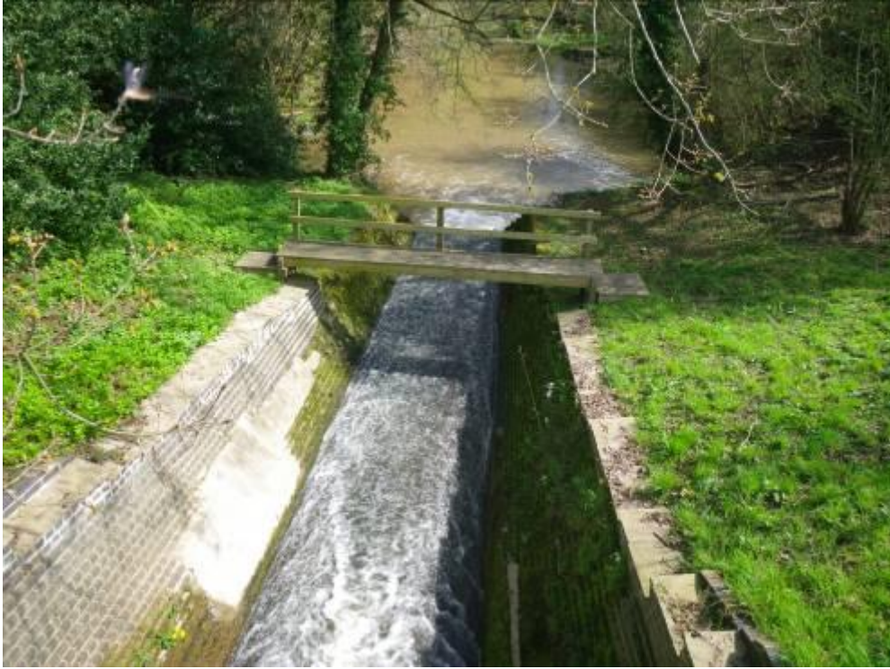
Photo 5. Downstream end of existing outlet – a high velocity chute.
