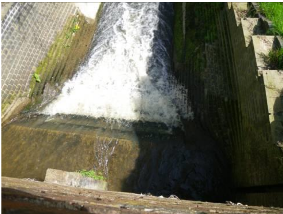
Photo 4. Existing outlet structure. No options for fish passage at this location.
