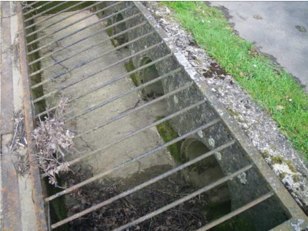
Photo 10. The inlet side of the spillway.
