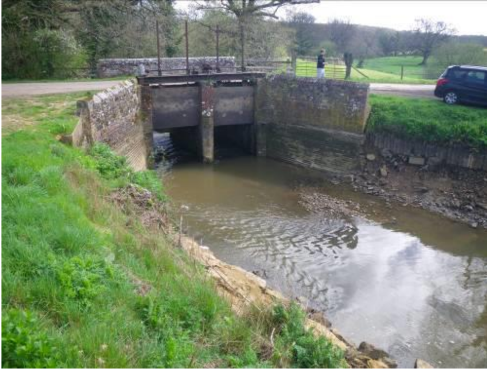
Photo 1. Existing pond outlet. If the river channel were to be restored, the hatches could be removed and this channel left as an emergency spillway with no operational requirement or maintenance liabilities.
