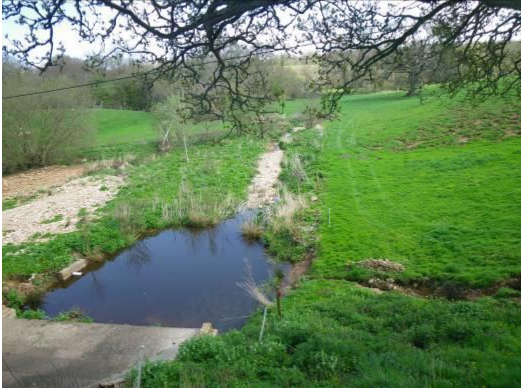
Photo 9. Spillway channel. Potentially the route for a new main channel.
