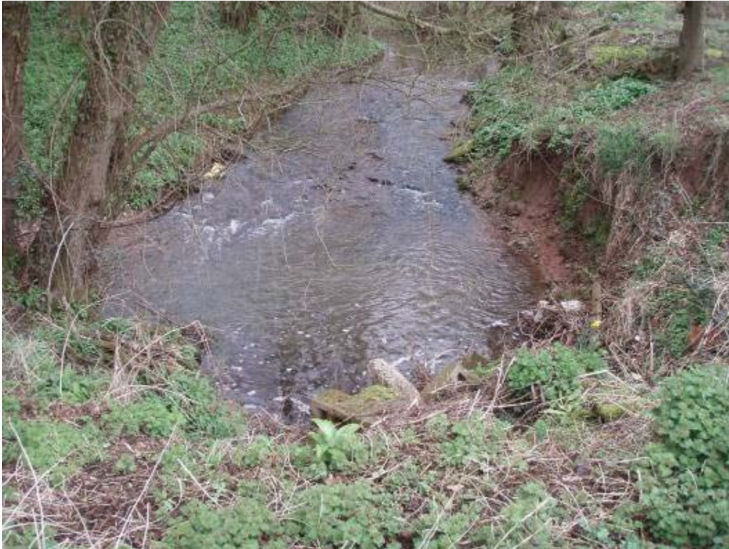
Photo 12 Area where a tree has been lost and the bank has become scalloped. Building waste has been tipped here to slow erosion but is unlikely to be effective.
