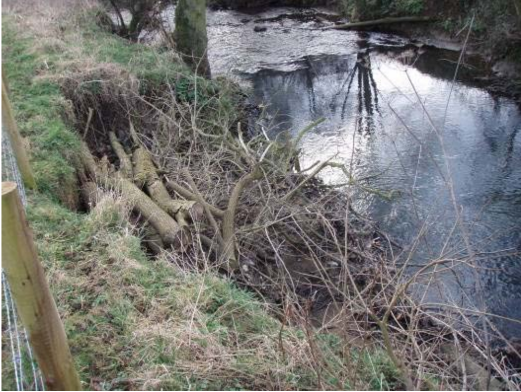
Photo 13 Example of brushwood packed into a scalloped bank and wired in place, then fenced out. The bank here has since accumulated sediment and consolidated (River Ecclesbourne, Derbyshire).
