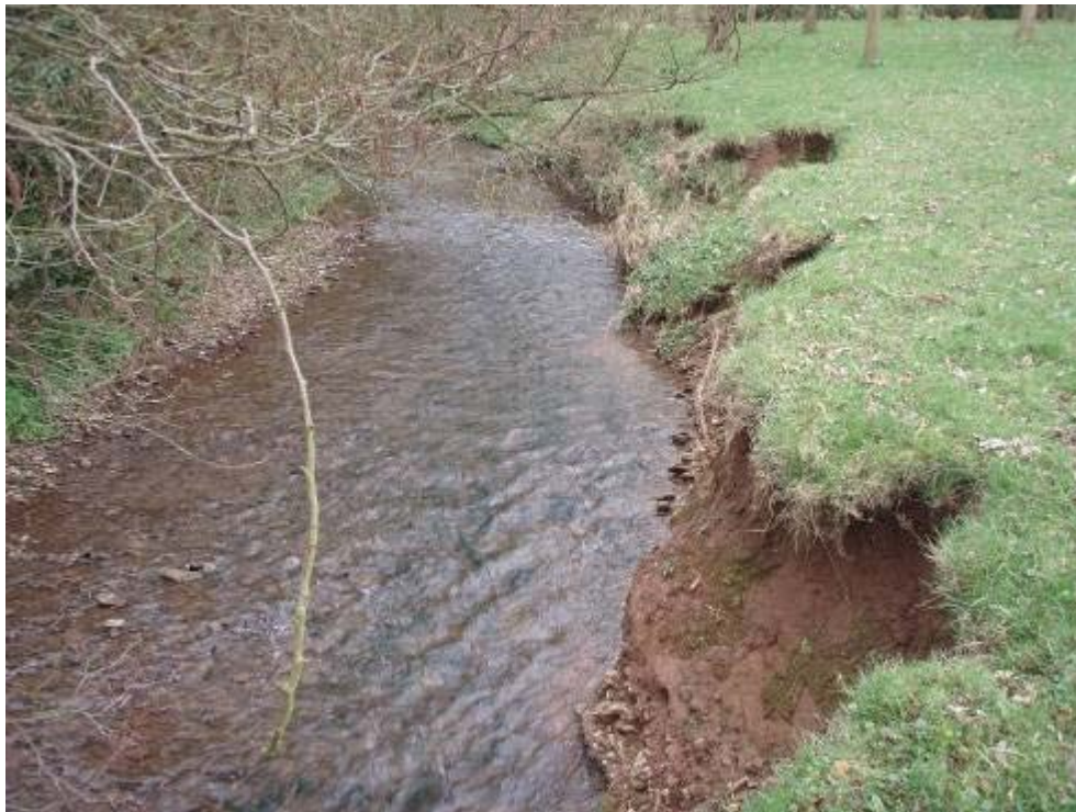
Photo 4 Grazed banks erode easily leading to over-wide, shallow channels with limited in-stream habitat value.
