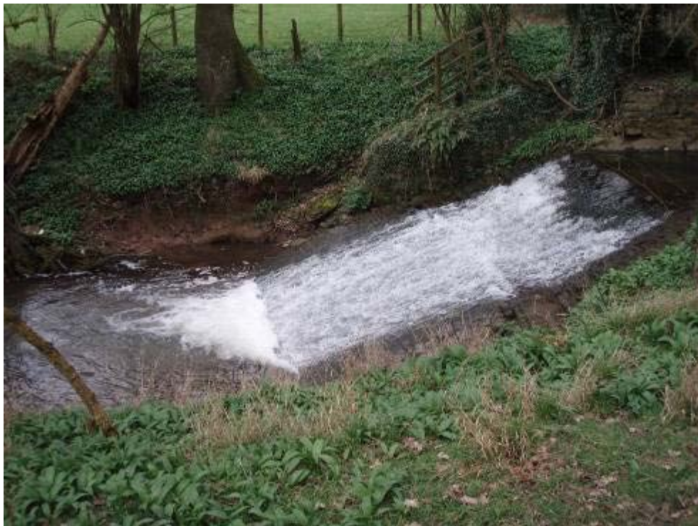
Photo 1 Weir at the upstream extent of the reach
