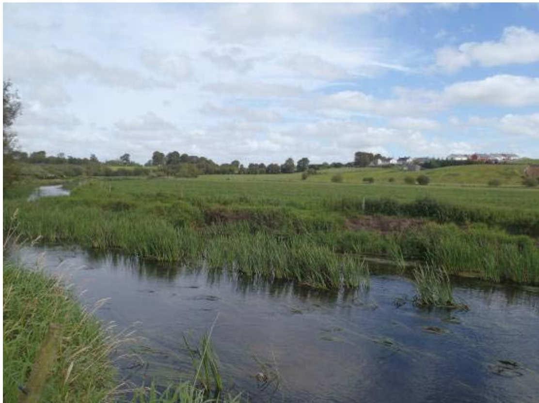
Typical length of the Little Brosna showing eroded bank and resulting emergent vegetation stands
