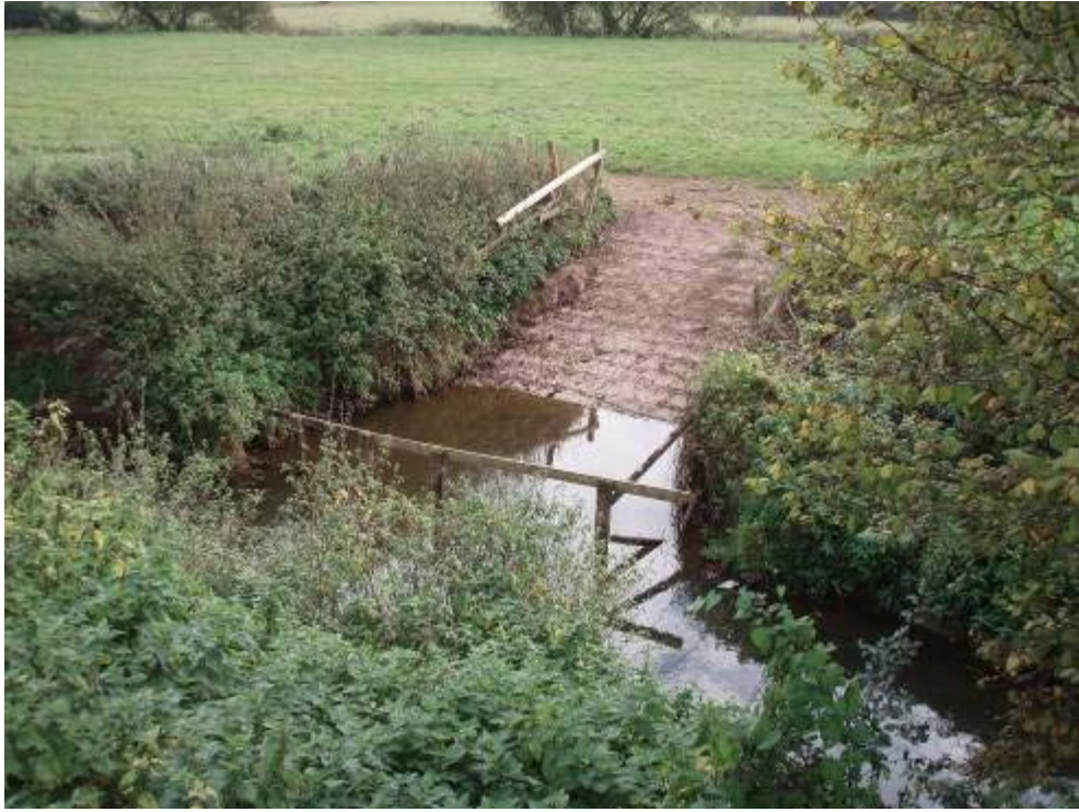
Photo 4 More formalised stock watering area on the LHB; the ramp is reinforced with concrete sleepers.
