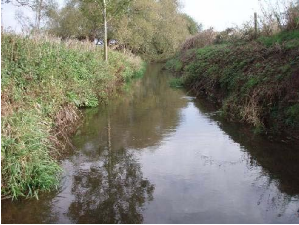
Photo 2 As above – a straightened, trapezoidal channel with steep banks and little variation in channel dimensions
