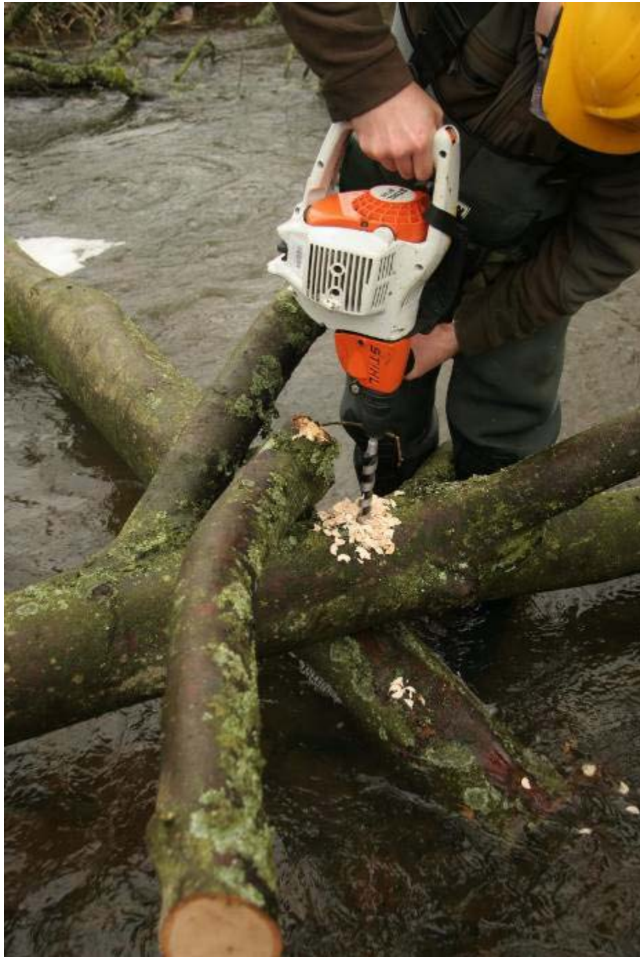
Photo 11 Using a wood auger to bore holes in LWD
