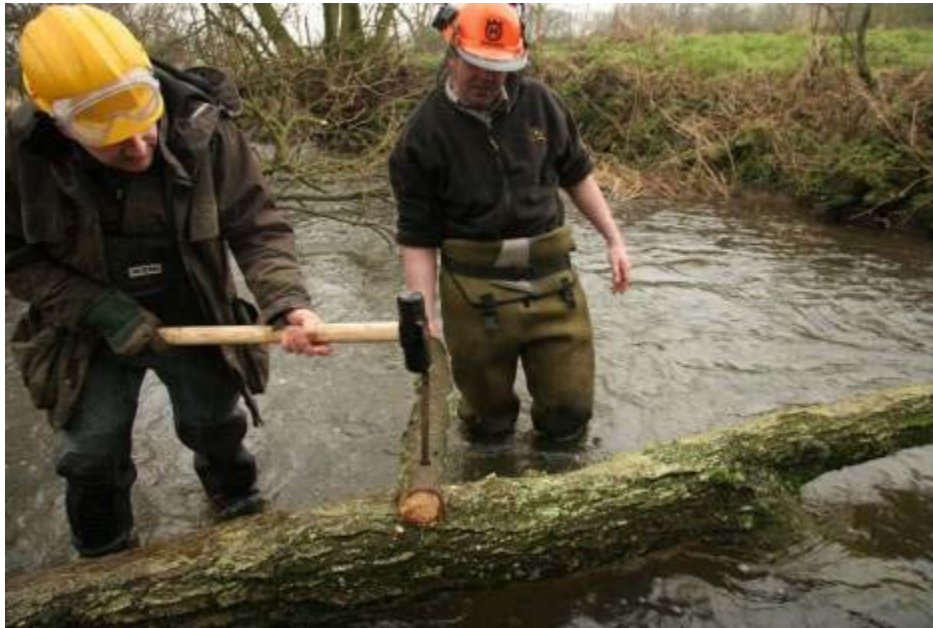
Photo 12 Fixing LWD in position with steel rebar
