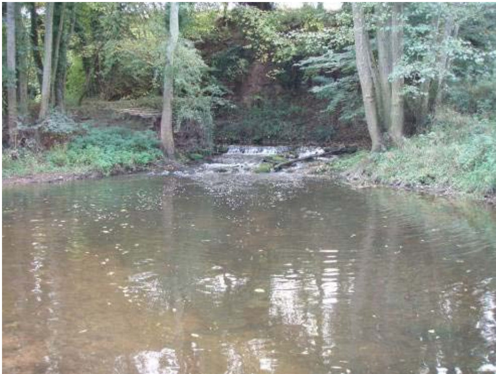
Photo 7 Old weir structure above Durbridge Mill
