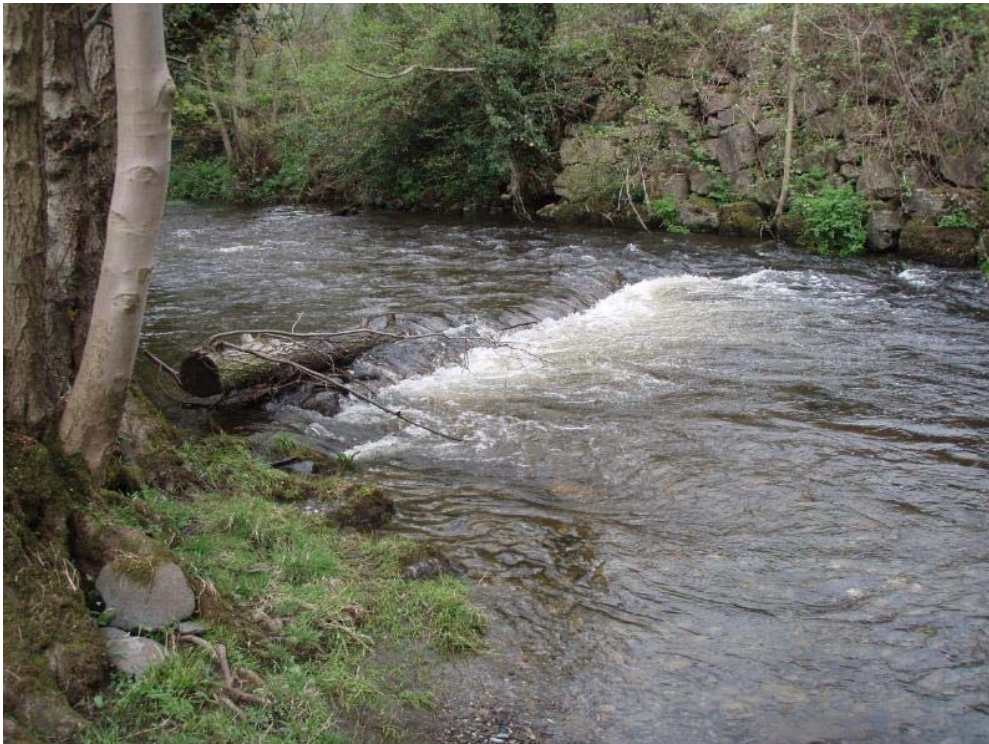
Photo 20 Large woody material pinned to the river bed to promote localised bed scour and depth variation.
