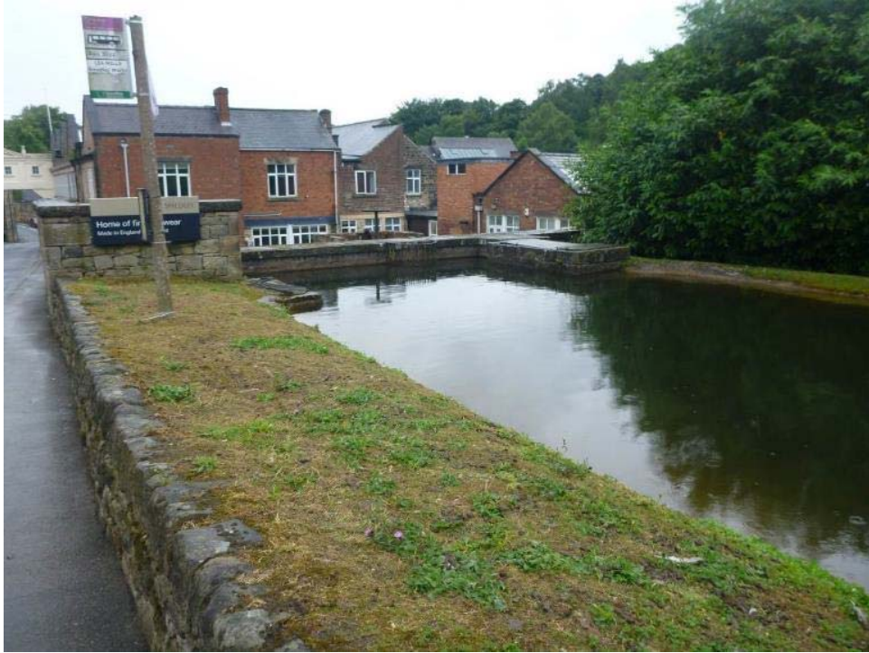
Photo 16 Reservoir located upstream of the factory which supplies water to the factory sprinkler system. The reservoir is topped up by a feed from the brook.
