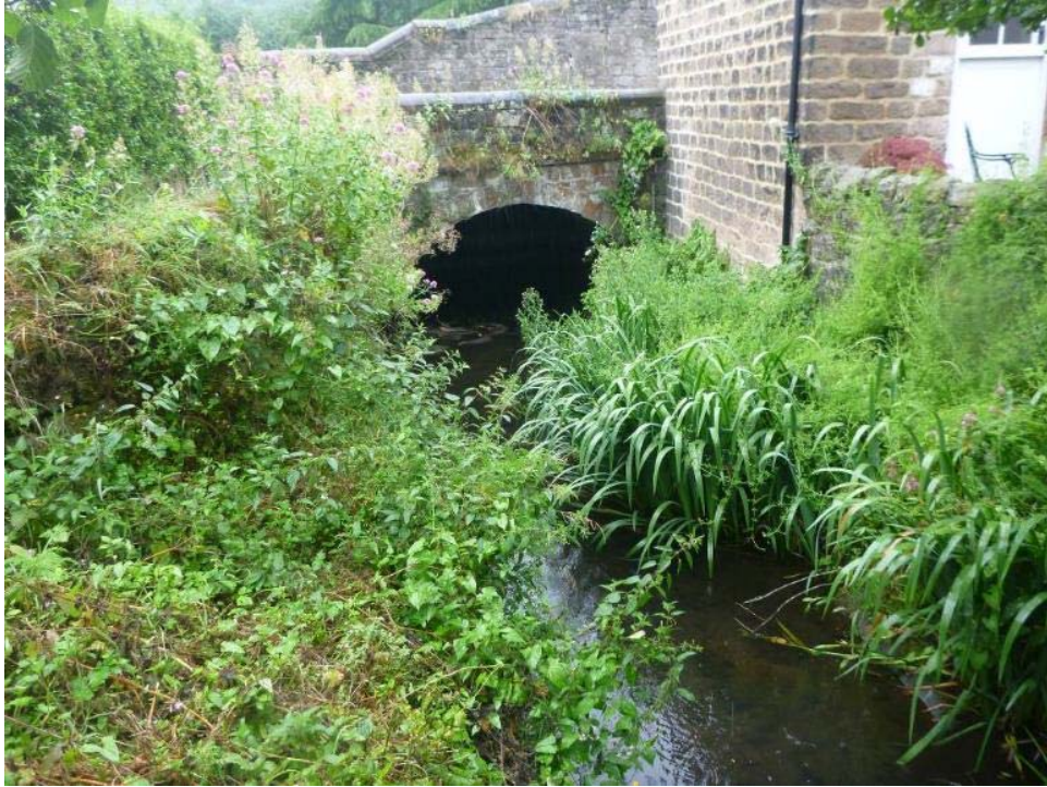
Photo 1 Bridge at the downstream end of the section.
