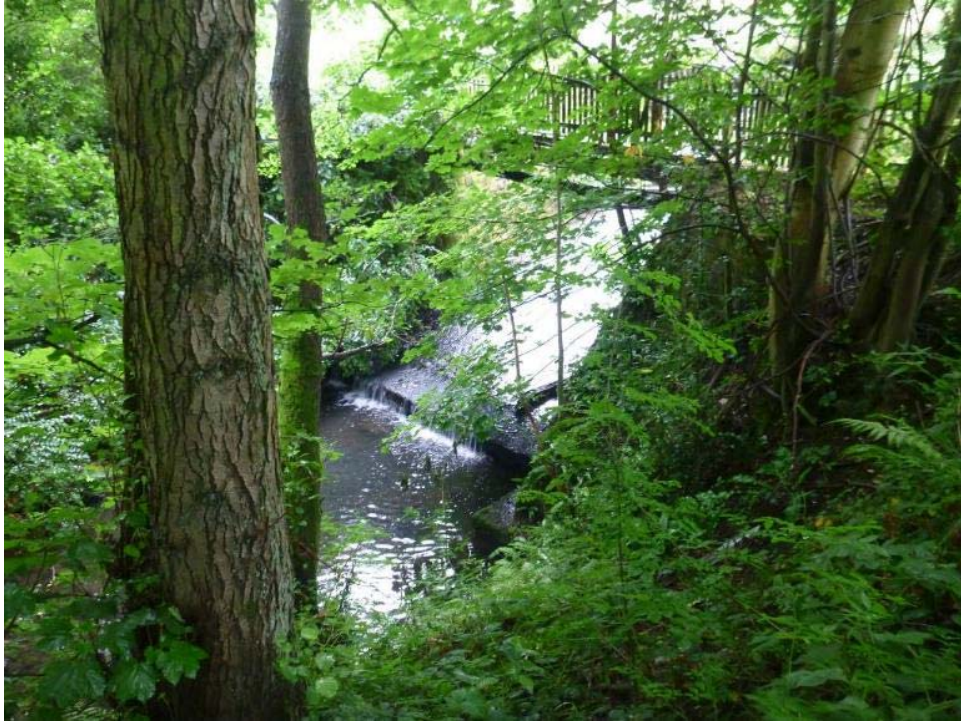
Photo 18 The downstream lip of the spillway of the above weir, beneath the footbridge. A trout was observed in the pool downstream but fish will not be able to ascend the weir structure in any flows, fragmenting the habitat of the brook.
