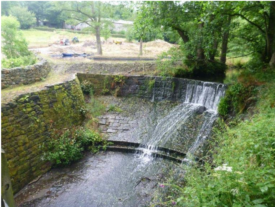
Photo 17 Large weir located on the brook upstream of the reservoir. The conduit channel to the reservoir leaves the brook on the LH bank (not visible, right of shot). A recently created pond is visible in the background on the site of a former mill pond.
