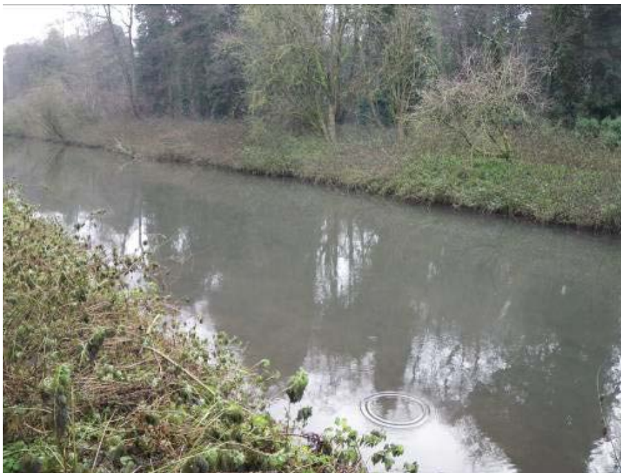
The top section of the beat where all the plants have been scraped out mechanically, destroying valuable habitat and not achieving an improvement to hydraulic conveyance.
