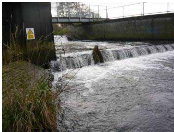
Flow gauging weir below Temple Bridge.
