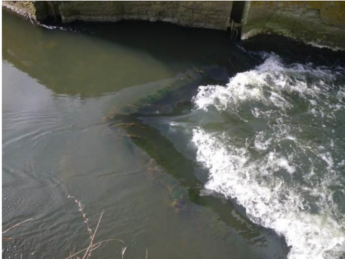
Photo 6. The old lock gate base impounds the reach upstream.
