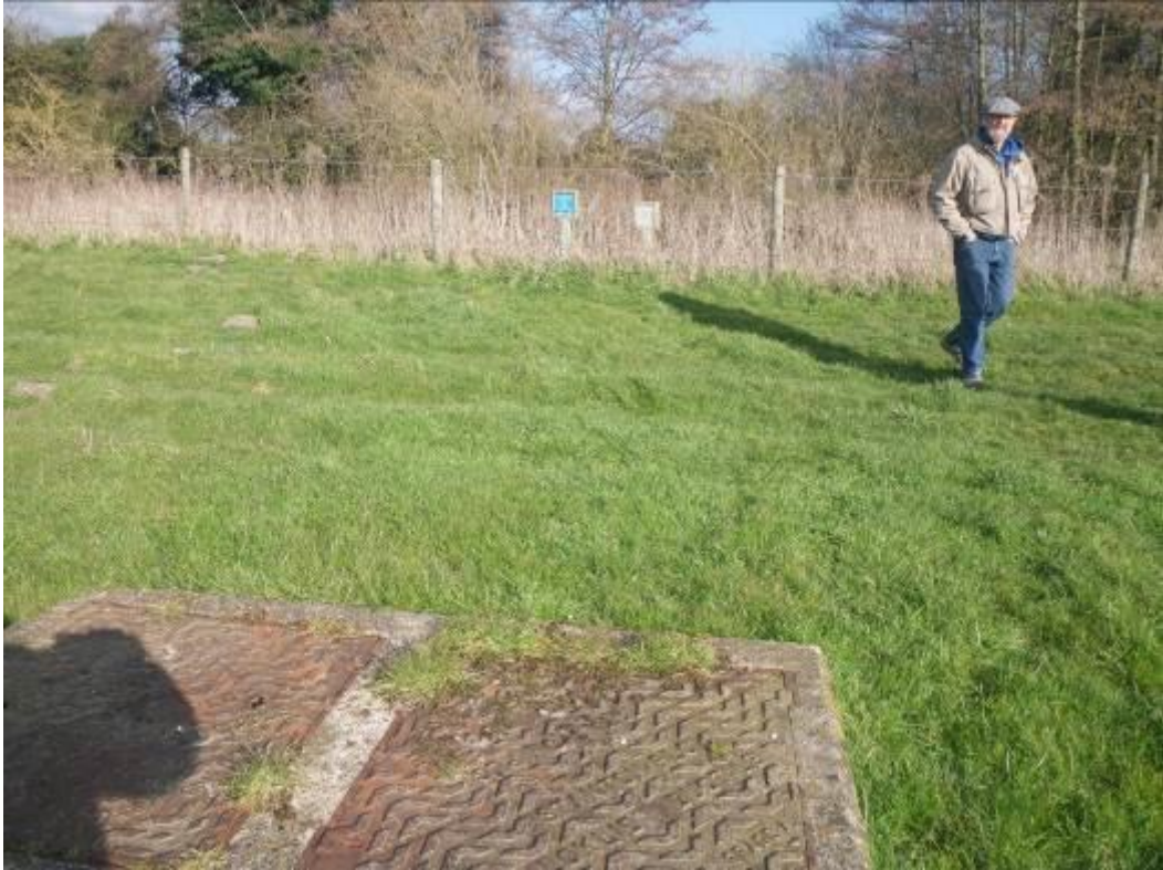
Photo 3 Large service crossing thought to be a trunk sewer.
