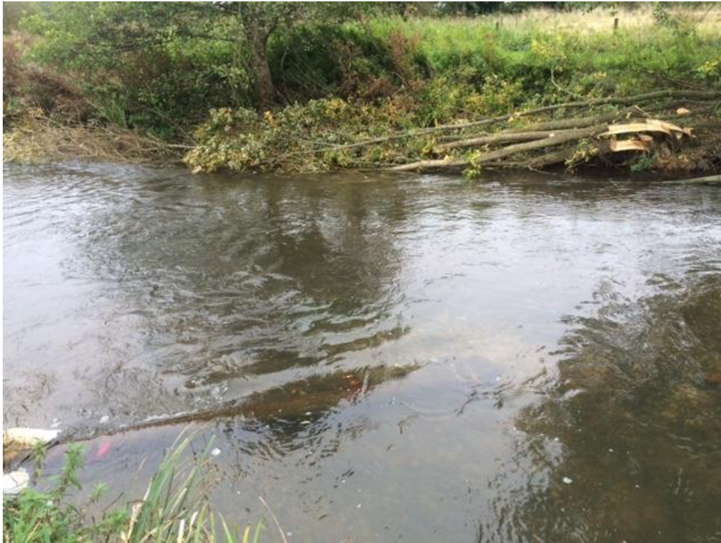
Photo 14. Log deflector combined with folded willow.
