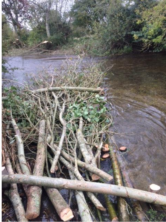
Photo 12. Brushwood mattress constructed with coppiced willow.
