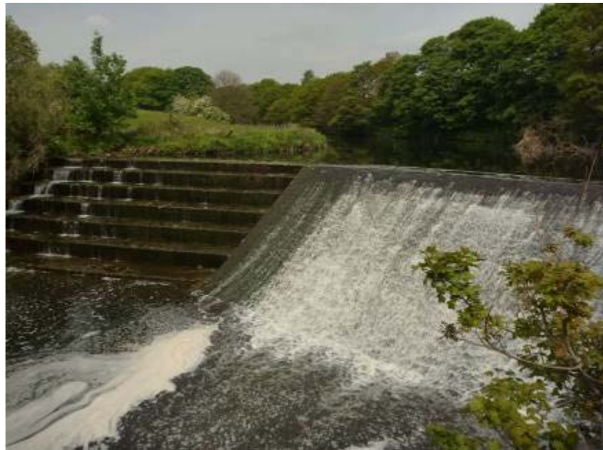
Figure 9: Weir with an estimated vertical head loss of ~25 feet at SD 79647 13073
