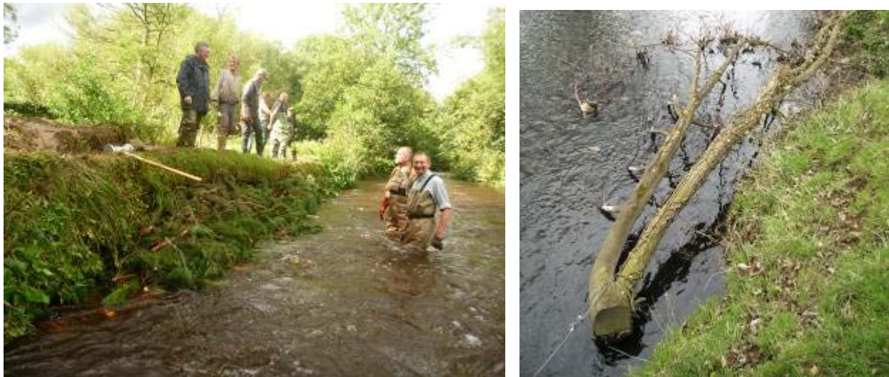
Figure 12: Marginal brush (L) and tree kicker (R) examples of marginal cover installation
