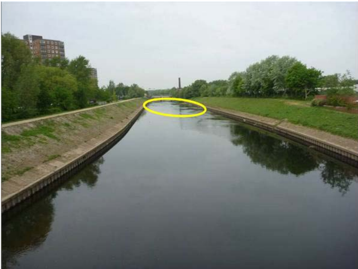
Figure 1: Engineered channel with old riverbed just visible (ringed) under low flow conditions during visit
