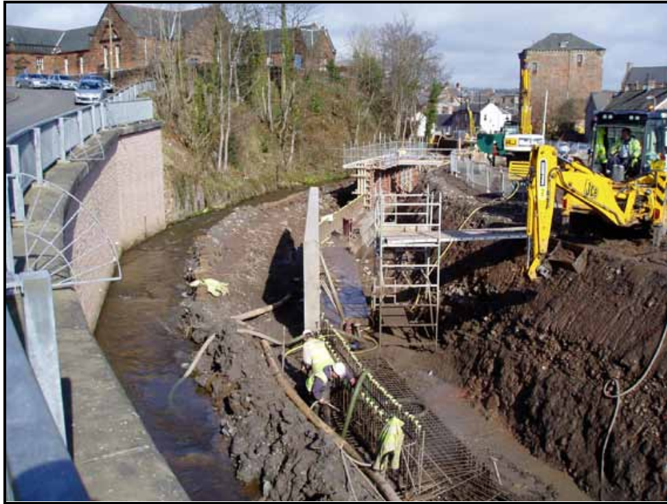
Plate II: Burnawn flood prevention works in Galston
