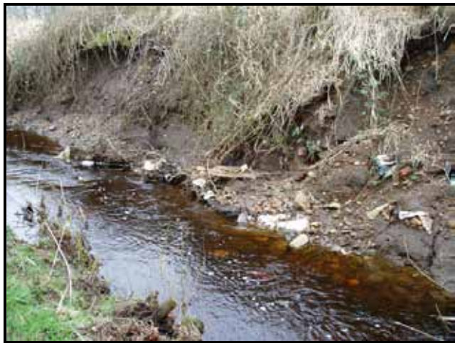
Plate XVI: Landfill material eroding into the burn
