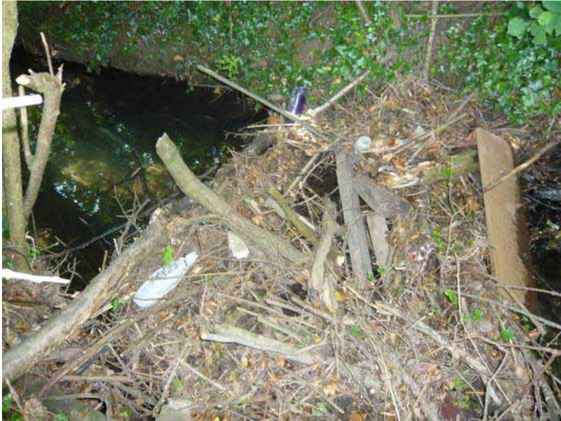
Debris dam on the Honeybridge stream
