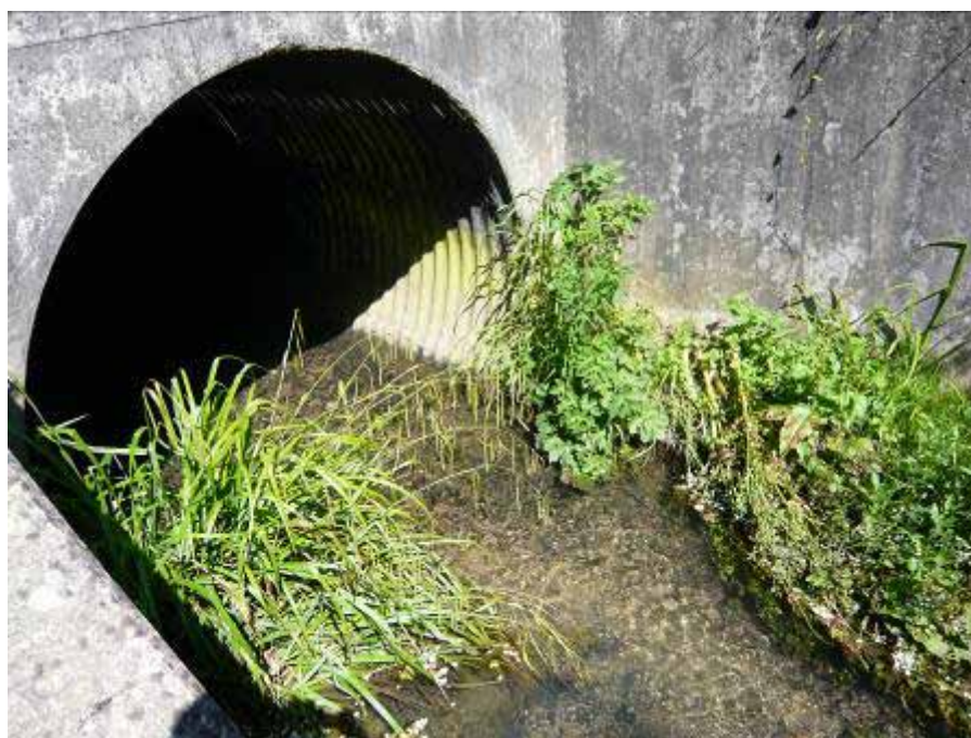
Culvert under the A24 marking the top boundary
