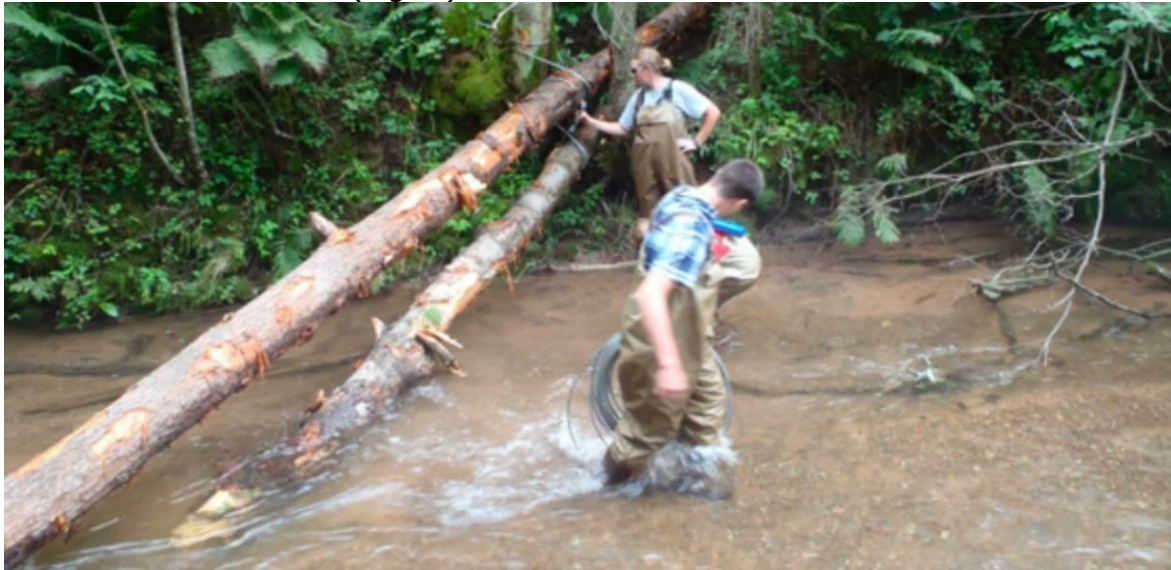
Figure 4: Illustration of how the angle of an individual log (here the picture includes two logs) from high on the bank provides clearance between the underside of the timber and the riverbed during spate flows. The length of timber on the bank can be much shorter (e.g. flush with the anchor tree). NB this is not an illustration of anchoring methods or proposed lengths of timber.
