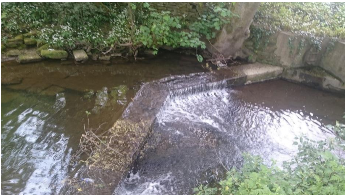
Figure 10: Low weir at SK 35866 70287. Sited on bedrock – so there is more limited potential for structural issues arising from removal at this point.
