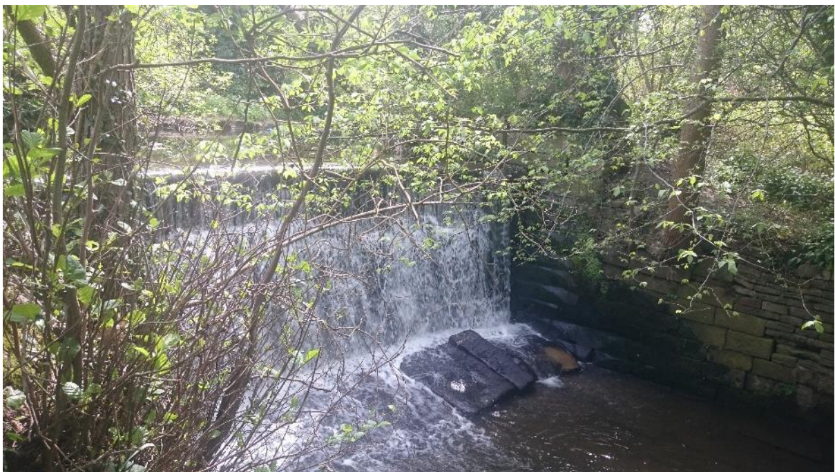
Figure 7: Huge weir relative to channel size at SK 35861 70273. This is less than ~20m upstream from the weir pictured in Fig. 5. It is located just downstream of the pronounced bend and wide pool in the middle of Fig. 1 and feeds a reservoir via a (partially-culverted) leat. As well as its ongoing function of feeding the reservoir, the removal of this structure is complicated by the likelihood of significant changes to the path of the upstream and downstream channels.
