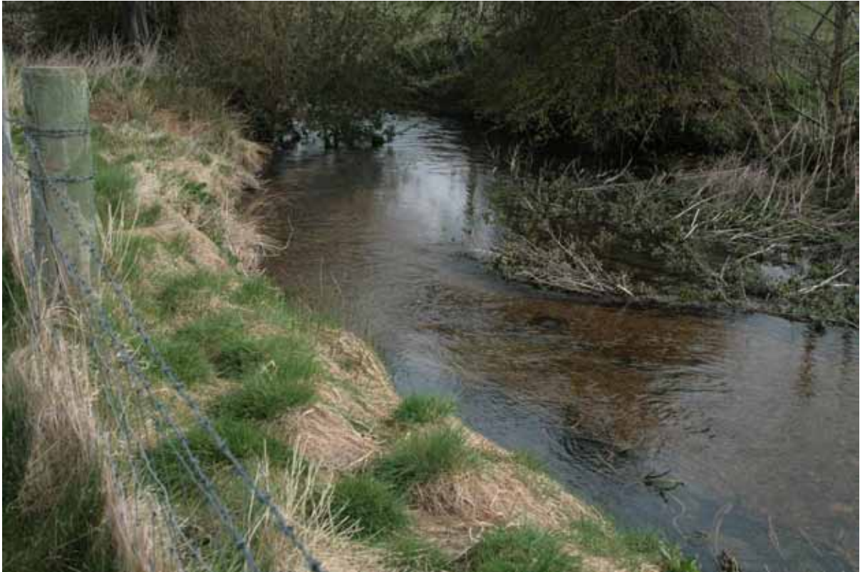
Formation of berm on inside of bend which is scouring silt and exposing gravels.
