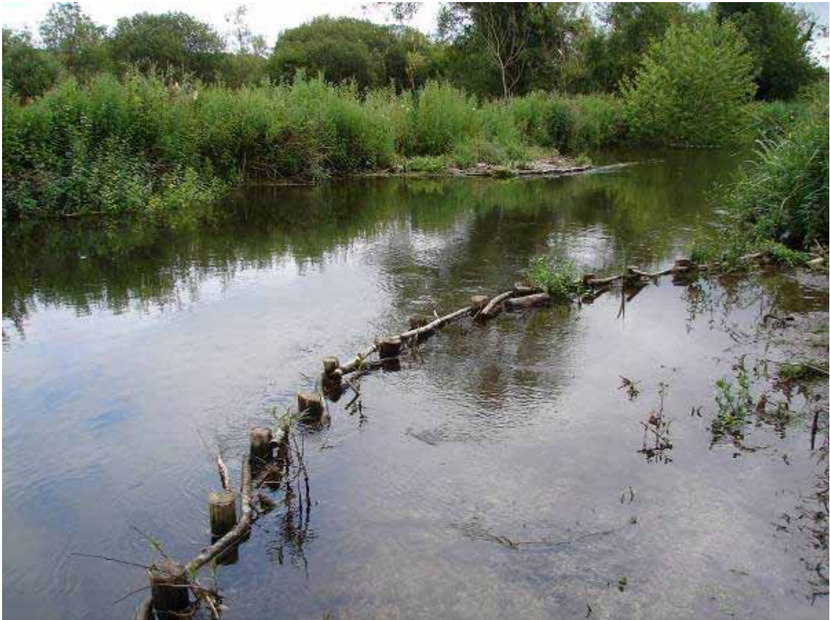
Example of spilling used to narrow both banks of the River Wylde, Langford – Wiltshire Wildlife Trust Reserve.
