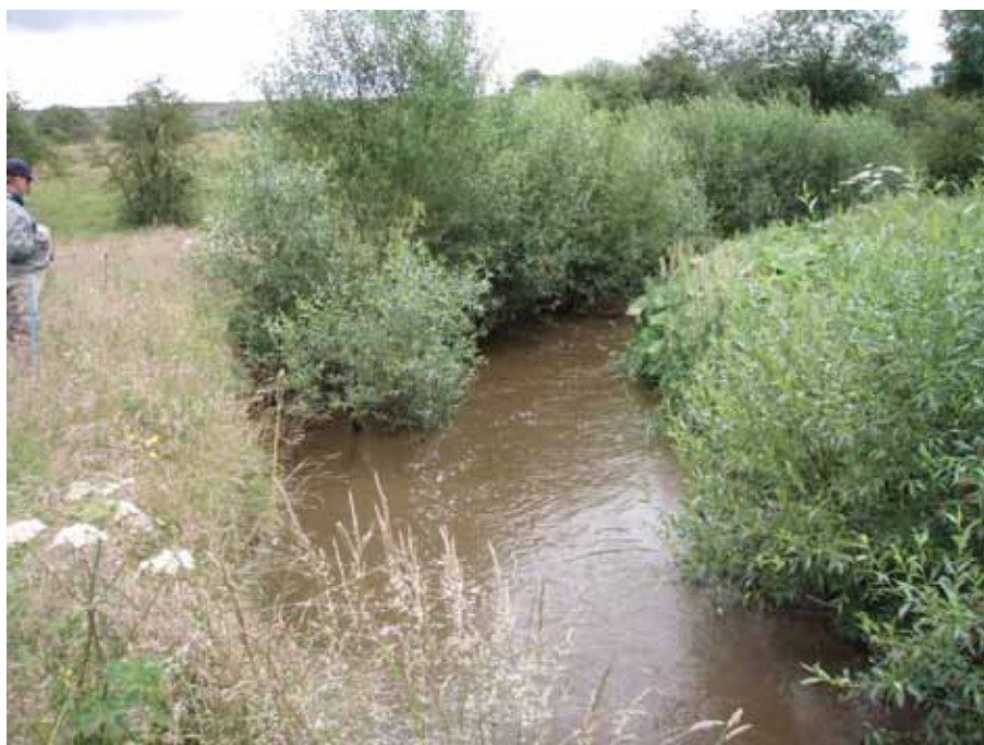
Photo 8 Willows planted on the outside of the bend and protected by electric fencing to arrest erosion
