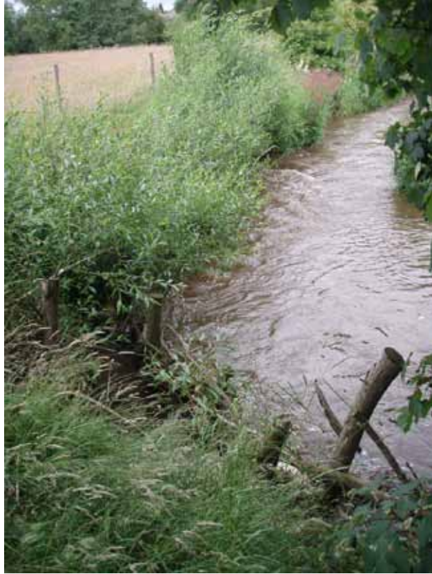
Photo 5 Willow spiling on right bank upstream of Papermill Farm
