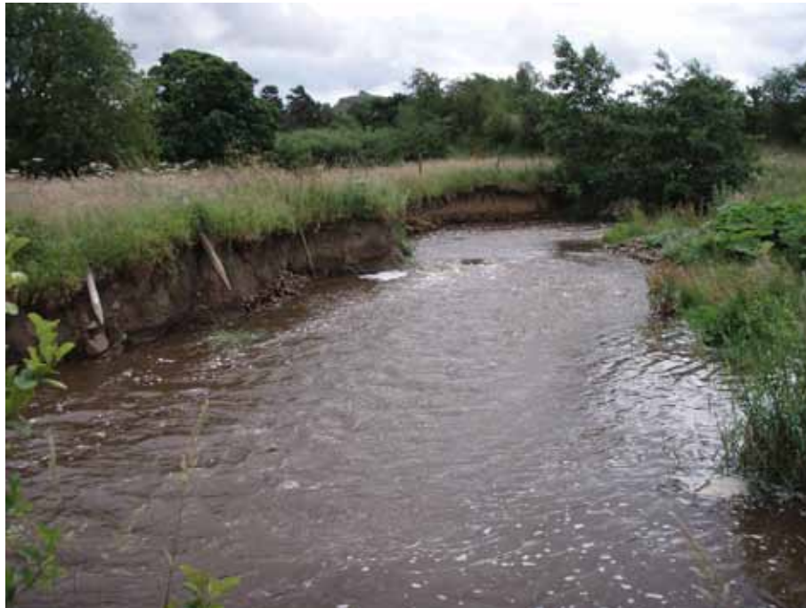
Photo 14 Area of rapidly eroding bank
