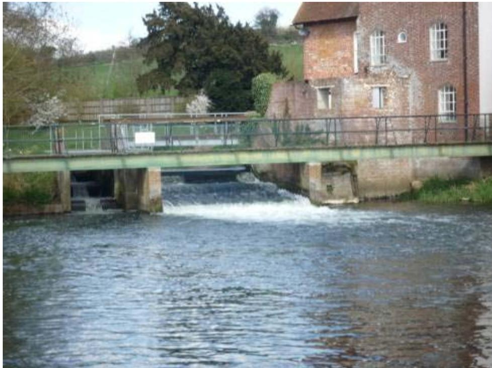
Weir pool forming the top boundary of the fishery. The attractant flow from the fish pass appears to be extremely low and will affect the efficiency of the pass.
