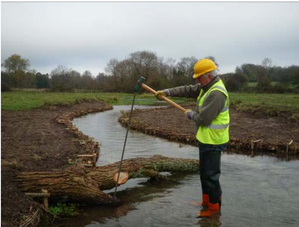
Installing an “undershot” LWD flow deflector on a Hampshire chalk stream
