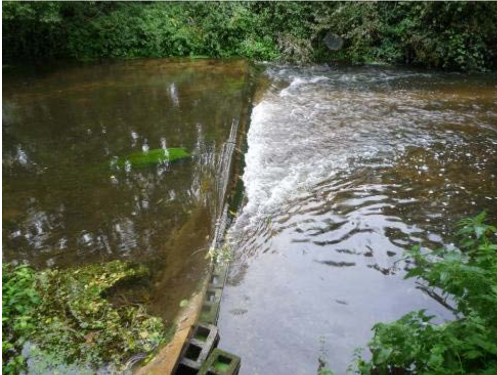
Block and slab low weir
