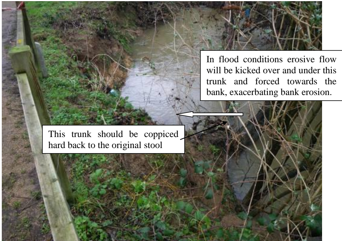
Photo 3. View from upstream looking down highlights the angle of the left hand trunk promoting the bank erosion.
