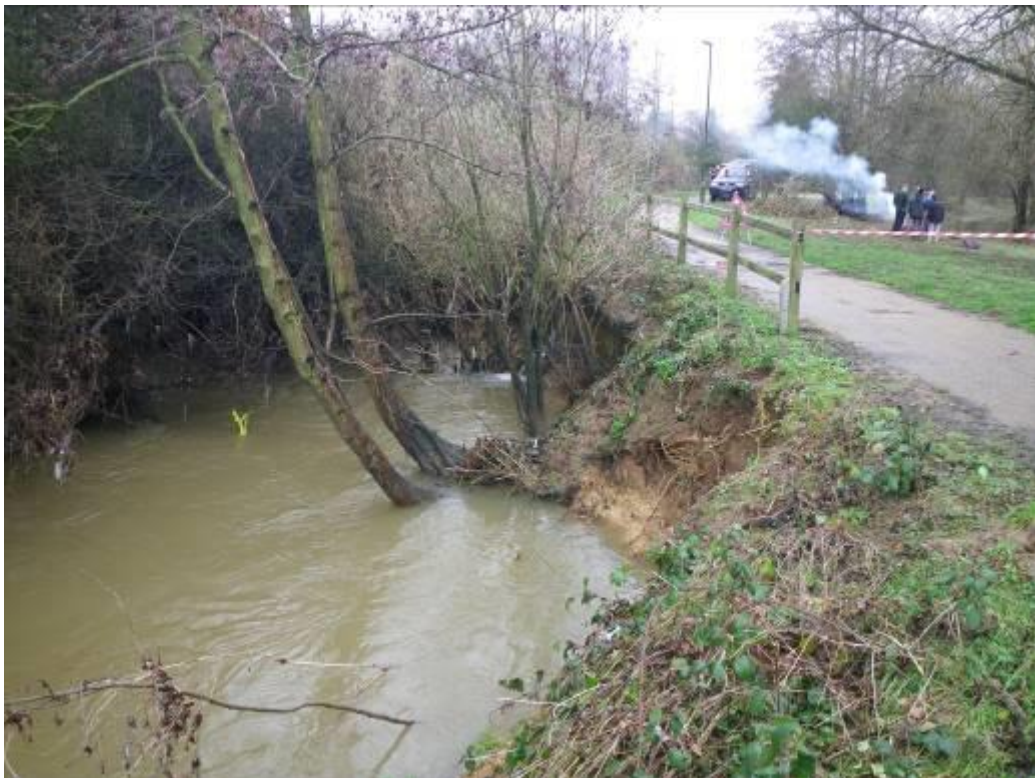
Photo 2 Another area where the path is in danger. Unfortunately the shape of the alders is forcing water into the bank under high flow conditions.
