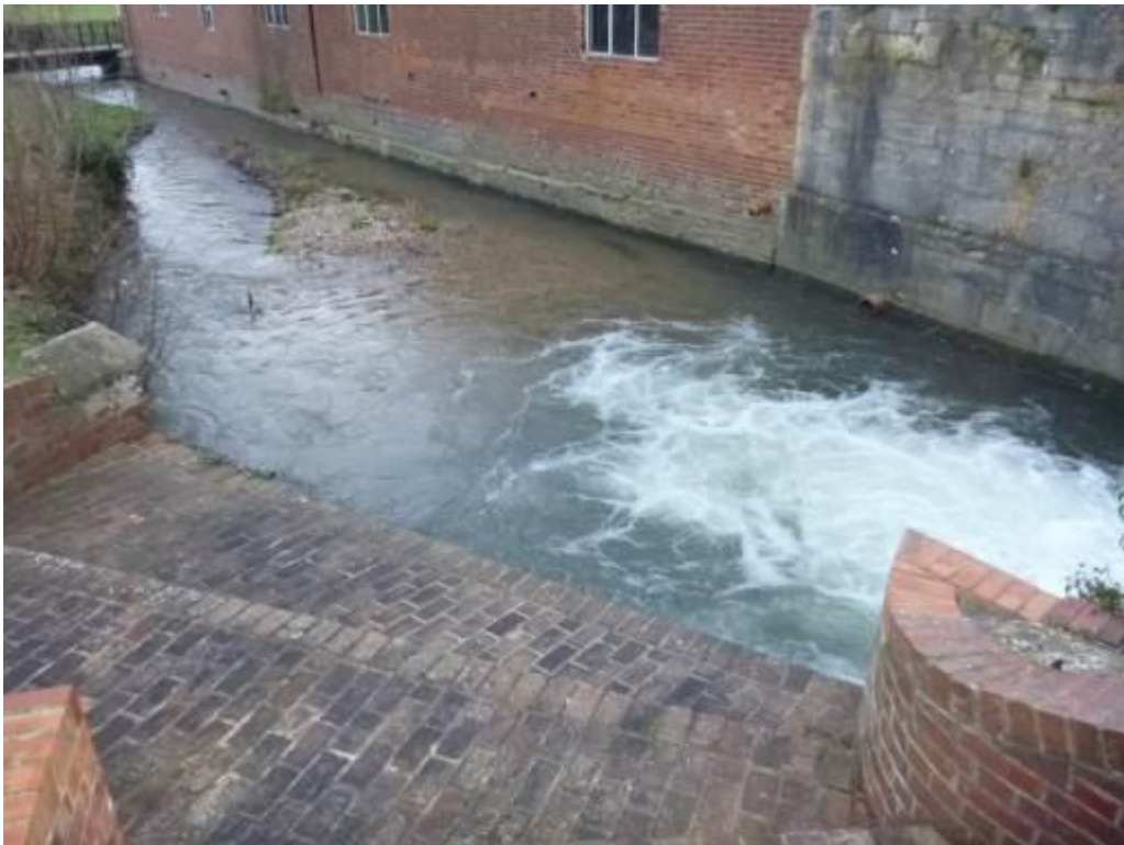
Photo 13 Weir into south channel adjacent to structure in Photo 12. Note gravel bed substrate.
