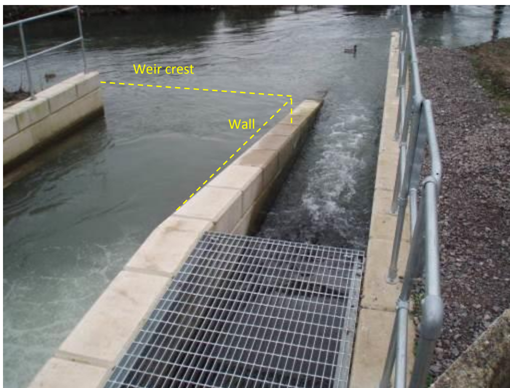
Photo 26 Locating the downstream end of the pass alongside the weir face, with a suitable retaining wall (as indicated by yellow lines) greatly improves pass efficiency. This should be considered at other sites.
