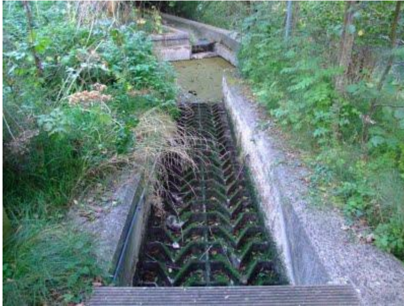
Photo 27 Example of a 1.2-m wide Larinier fish pass showing the two adjacent sets of 0.6-m wide baffle units (direction of water flow away from camera).
