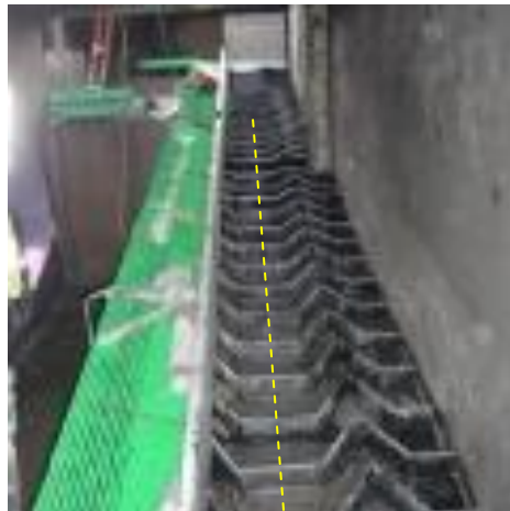
Photo 28 Example of one-and-a-half Larinier units plus angled bristle mat for eels (NB there should be a separator between the Larinier units in the position of the yellow line – as in Photo 18). Water flow towards camera.
