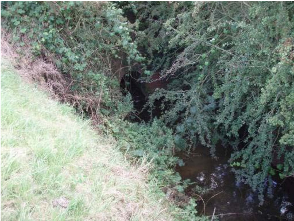
Photo 2 A culvert under the river channel carrying land drainage
