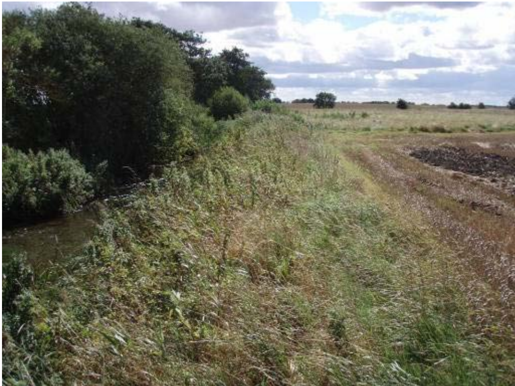
Photo 10 Looking downstream along the right bank – scope for re-profiling and pinching the river channel in places (see Photo 12).
