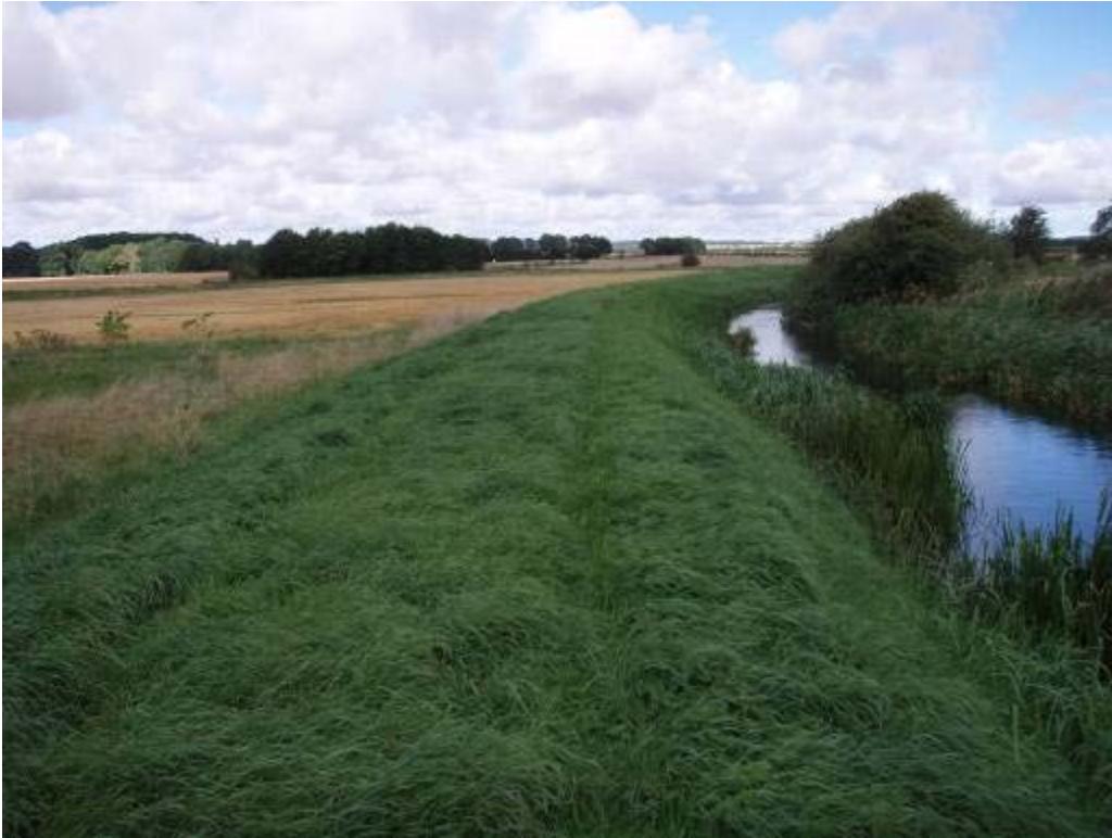
Photo 1 The Beck is in a perched channel above the level of land to the west (left of picture)
