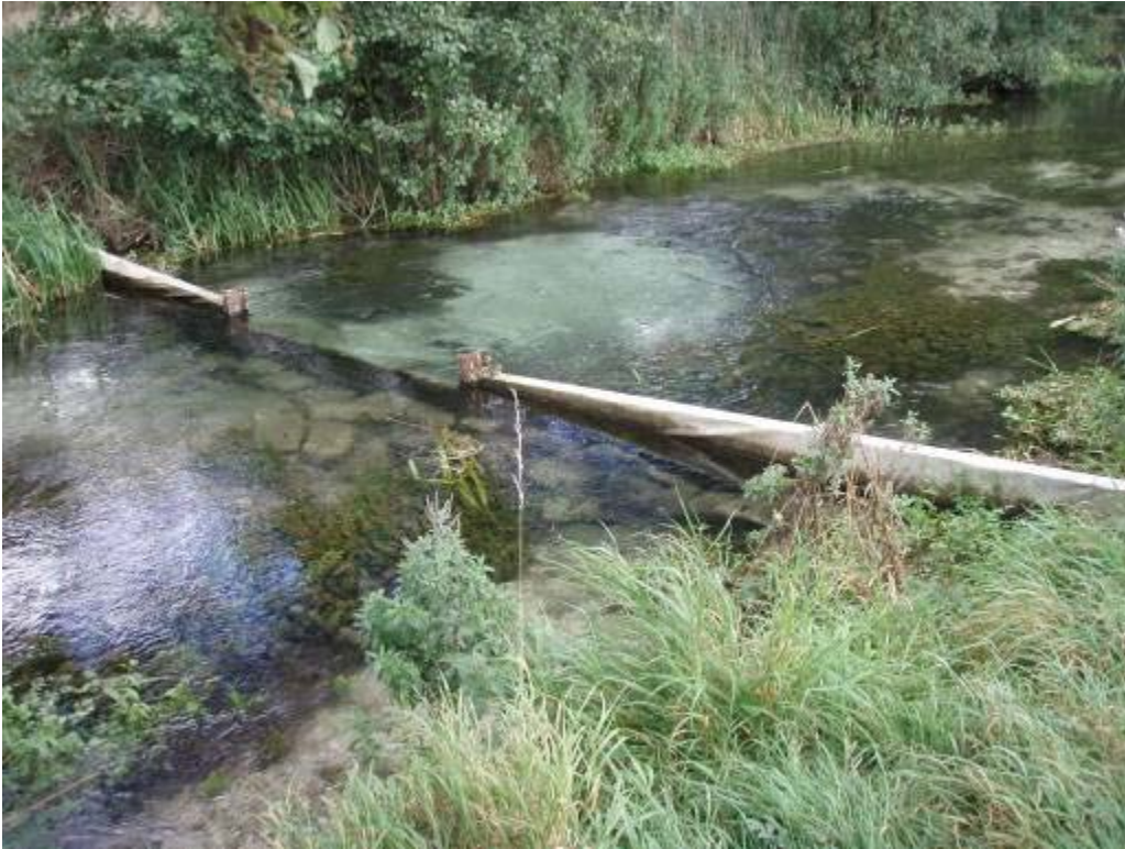
Photo 17 Weir downstream of Newroad Bridge showing removable boards and deep scour pool downstream
