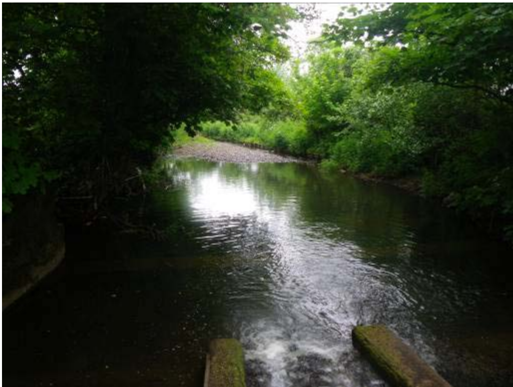
The Large gravel shoal may have been promoted by the installation of the fish pass
