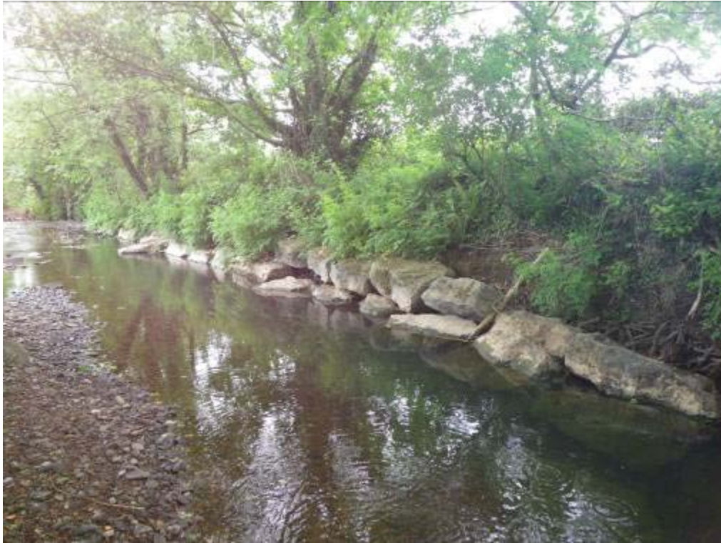
Stone revetment looks incongruous but will still be providing some cover for fish.
