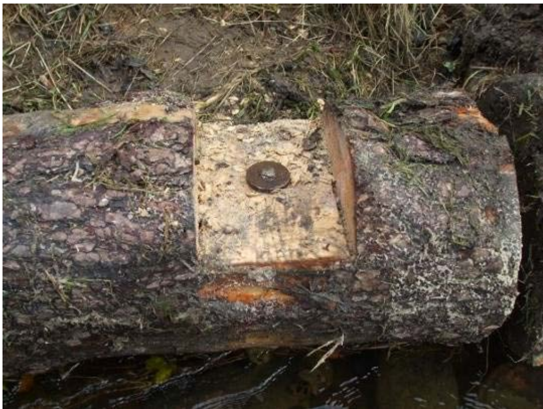
Alternative method for securing LWD using a large washer welded to 16-20mm rebar.
