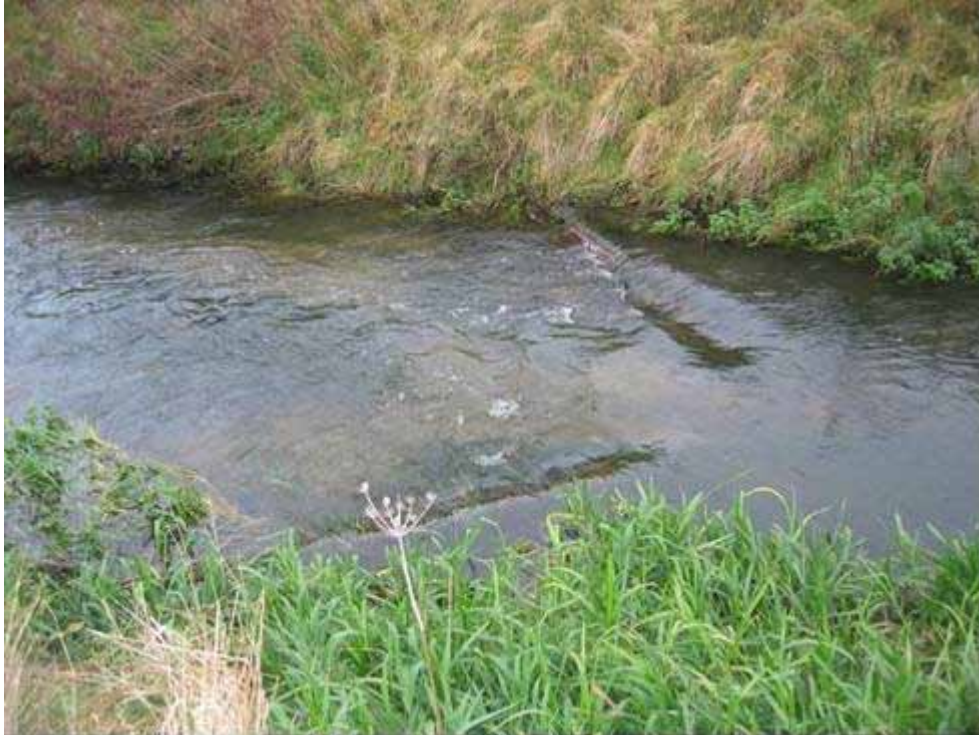
Photo 9 Paired flow deflectors scouring a deeper area in the centre of the channel – these could be used on the bypass channel.
