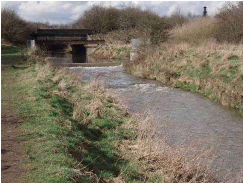
Photo 2 Overflow weir – view from bypass channel RHB
