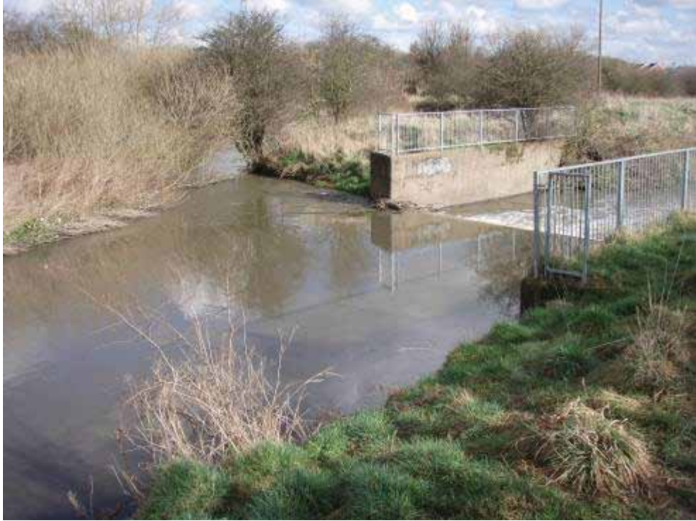
Photo 1 Overflow weir showing main river channel (left) and bypass channel (right)
