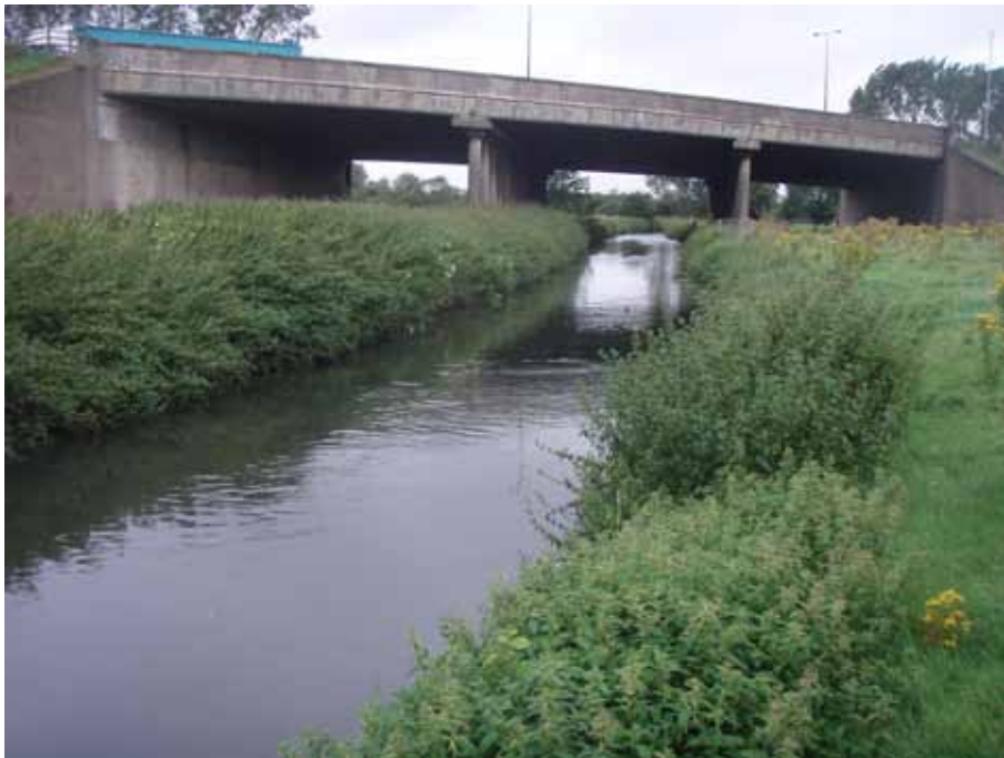
Photo 5 Straightened, concrete-lined channel under the M1 motorway.
