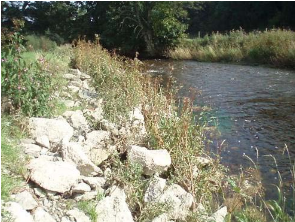
Photo 6 Concrete block rip-rap used to reinforce the river bank
