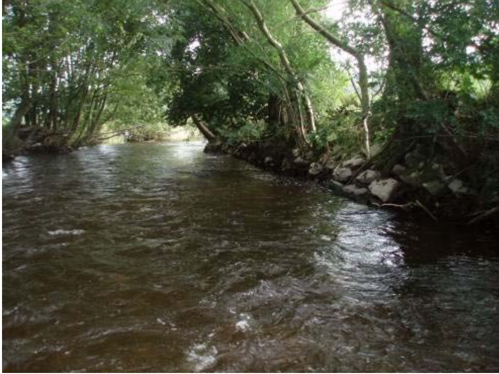
Photo 7 Older stone revetment with tree growth
