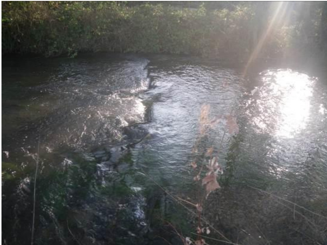
Photo 6. A low summer weir. The bed upstream has regraded and filled with small gravels and fine silt sediments. Removing a central block or two to the original bed level will improve habitat both above and below the structure
