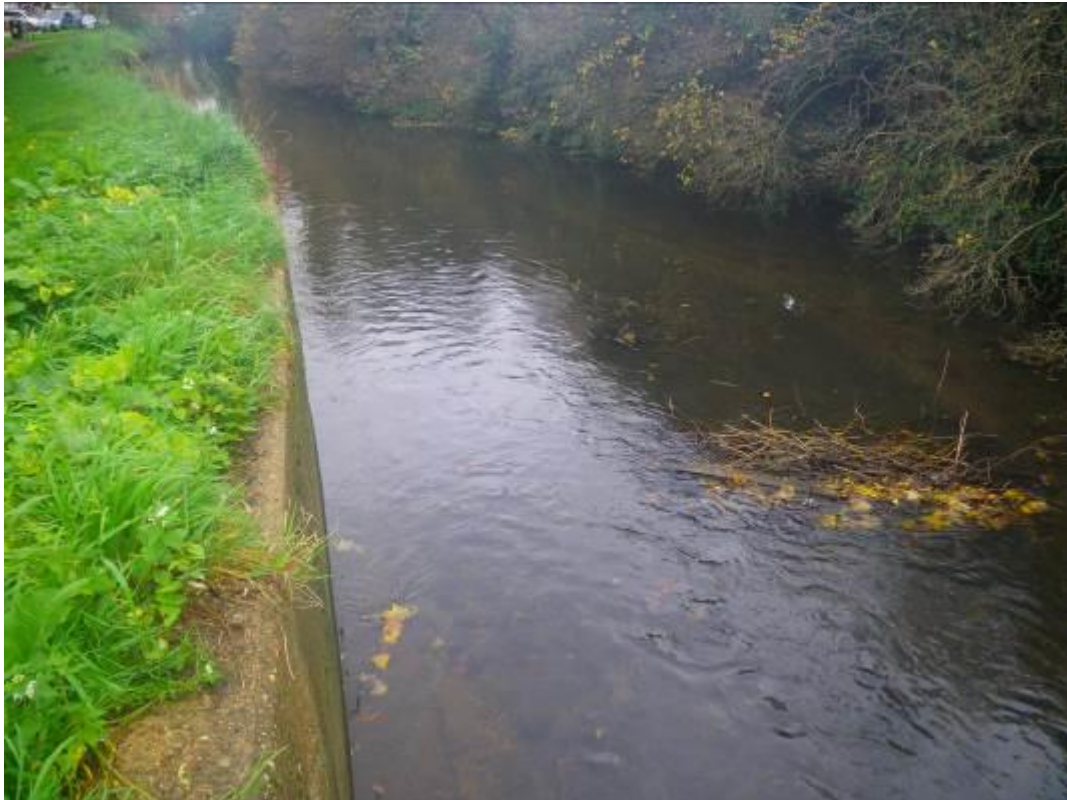
Photo 5. Biologically sterile concrete LB contrasts with the natural tree-lined RB, which provides some excellent habitat and resilient bank protection
