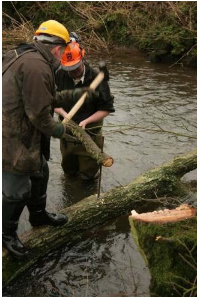
Photo 12 Installing LWD on the River Hamps
