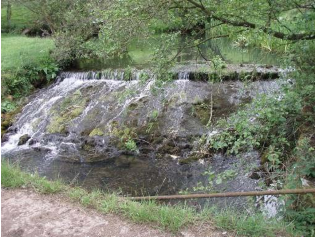
Photo 1 Weir adjacent to Ludwell Farm
