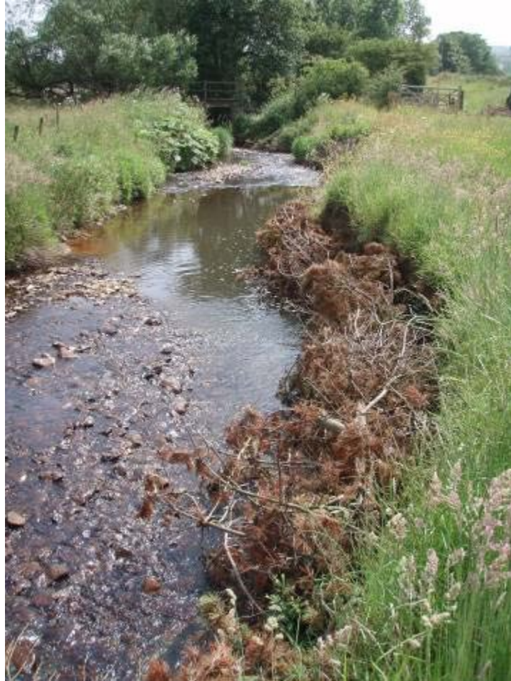
Photo 13 Soft revetment using brushwood on the River Manifold – this has provided excellent marginal cover for small trout as well as for riverfly species such as the southern iron blue.
