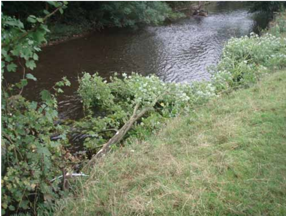
Photo 23 Whole tree anchored alongside the bank with steel cable to a standing tree (River Goyt, Cheshire)
