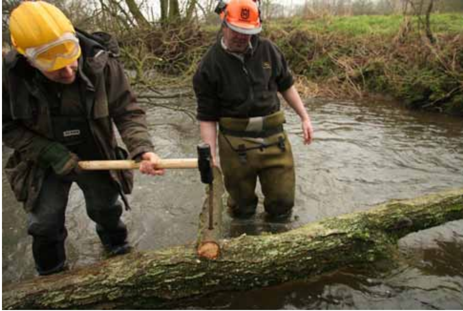
Photo 22 Fixing LWD in position with steel rebar
