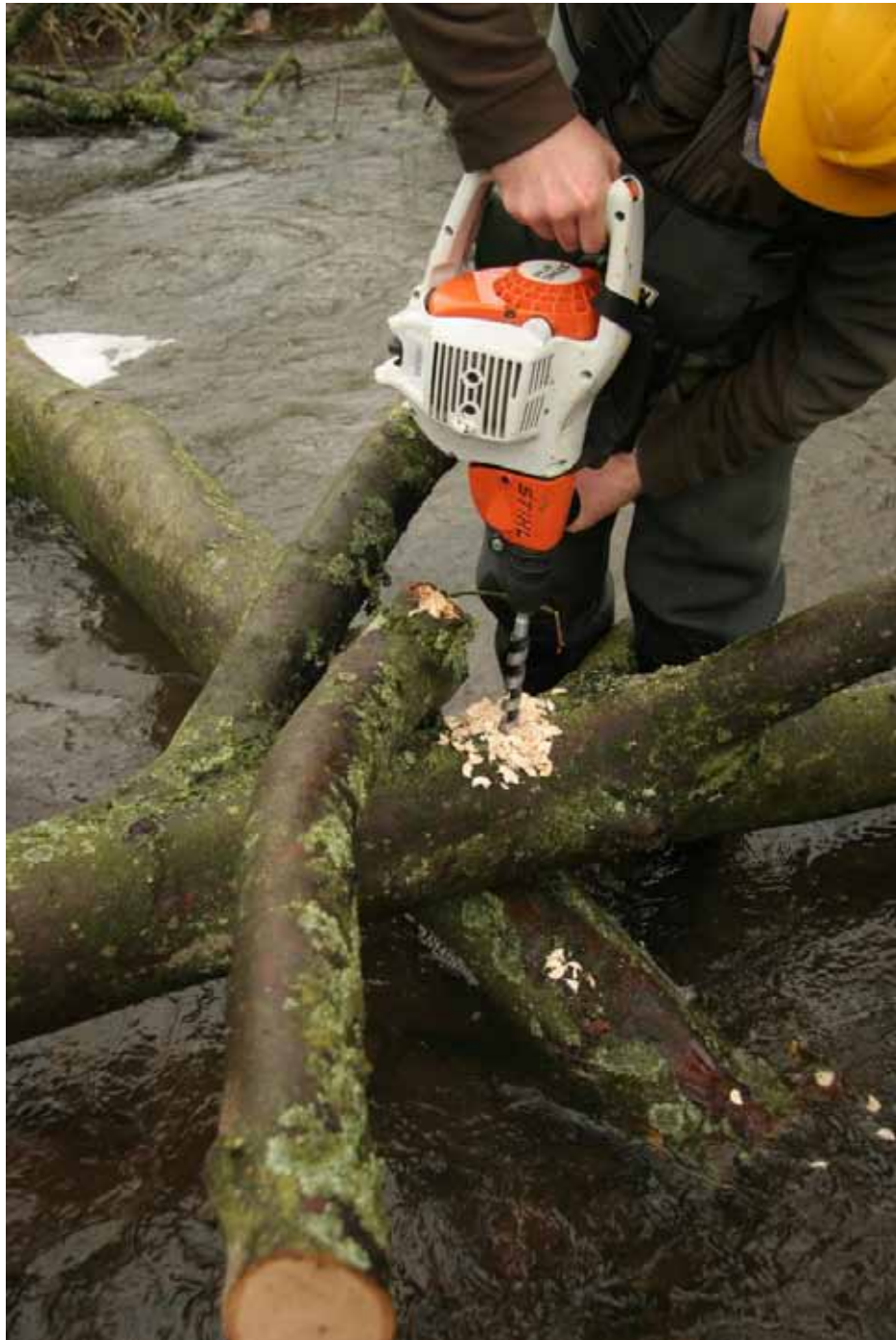
Photo 21 Using a wood auger to bore holes in LWD
