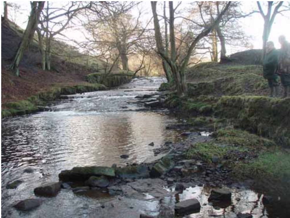
Photo 12 The weir constructed from block stone
