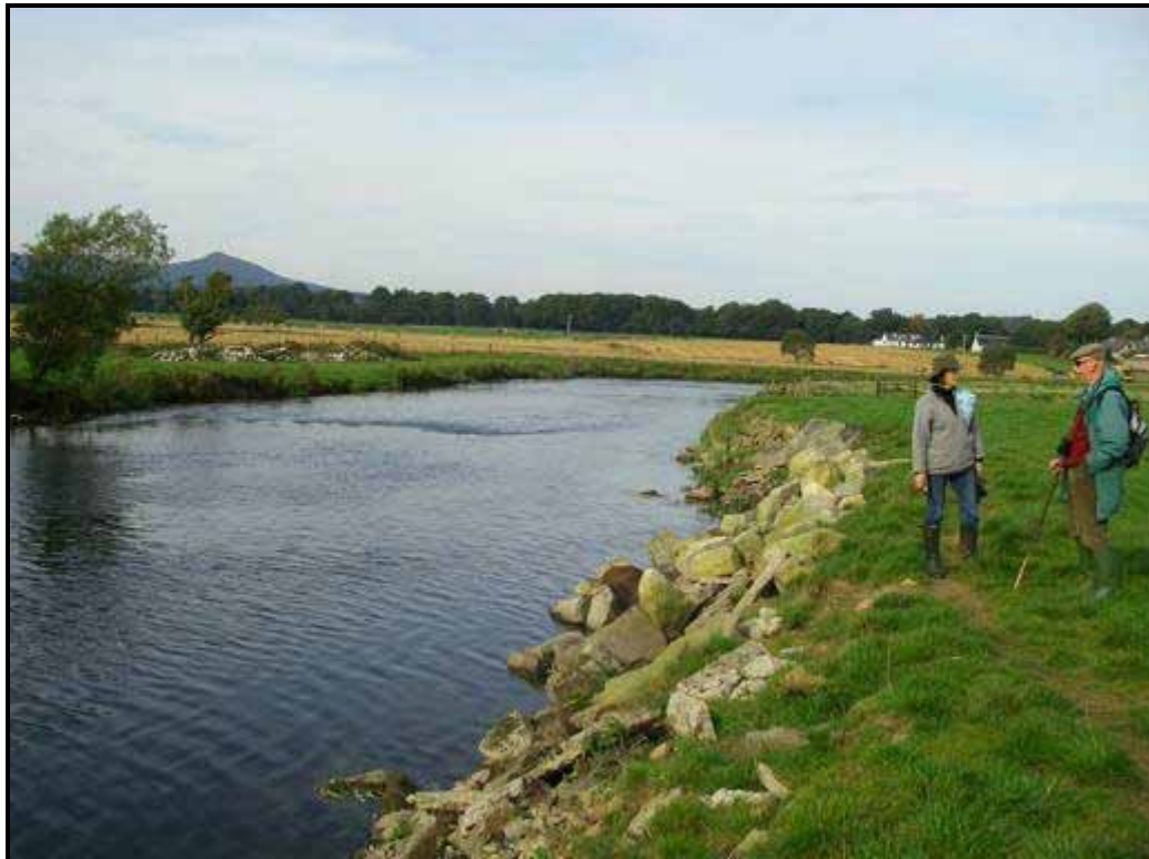
Plate V: Loose rock and concrete revetment materials which may have been dumped illegally on both sides of the river are only a temporary solution to bank erosion
