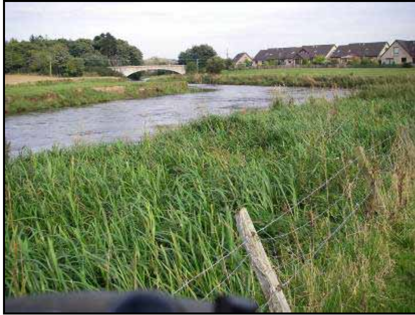
Plate VI: The positive effect of fencing to create a buffer zone of vegetation and provide protection against bank erosion is amply shown in the lower beat and on parts of the left bank (e.g. above Boatleys)
