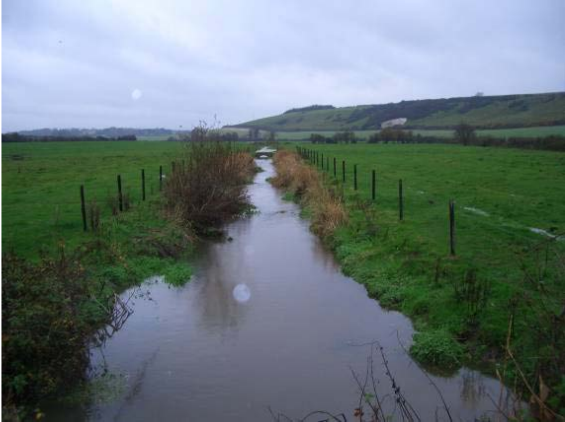
The top section of the Devils Brook has been realigned as a “drowning” carrier. The channel is crying out for a more natural channel morphology.
