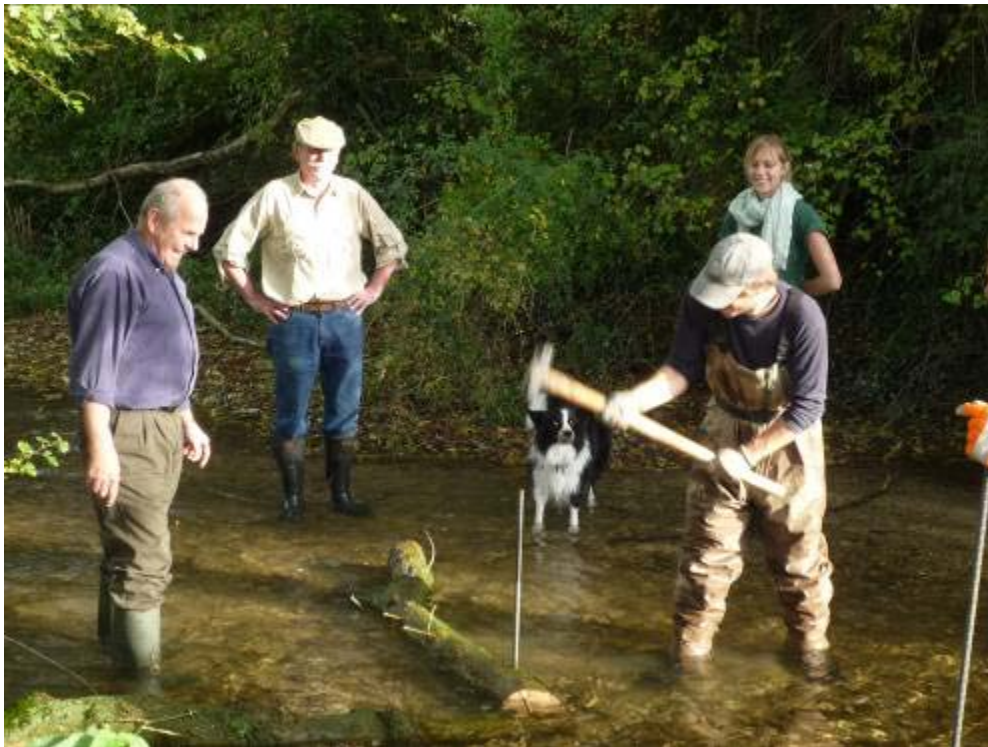
Pegging in a piece of LWD onto a shallow riffle on the Ebbles to promote improved spawning habitat
