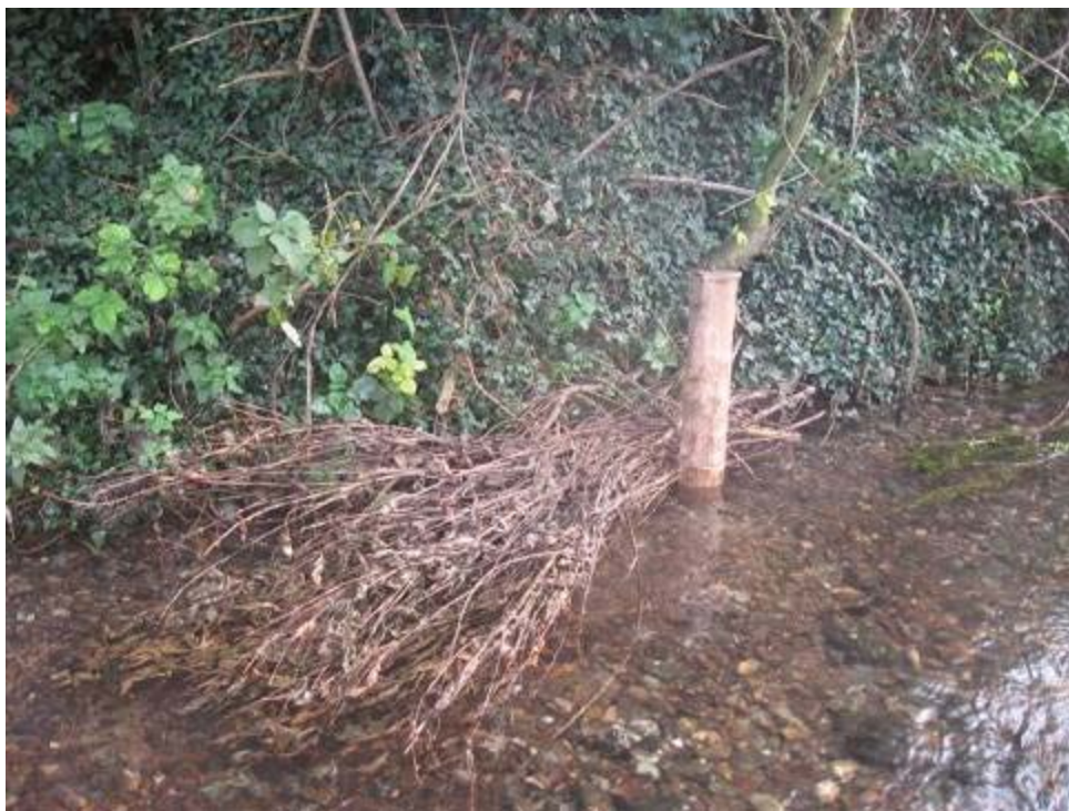
Brushings pegged into a bare shallow margin providing a refuge for juvenile trout
