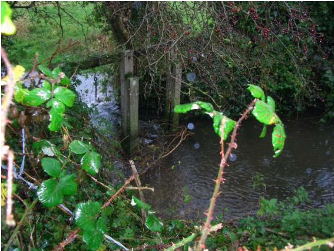
One of the numerous structures to be found on the Devils Brook
