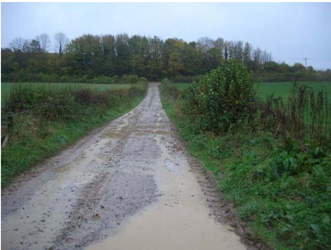
Track leading down to the Devils Brook acting as an arterial route for sediments running off the arable fields up behind the tree line.
