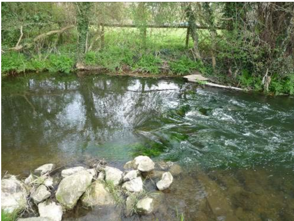
Old stone weir. Removing the central third of the weir will increase upstream water velocities and improve trout habitats
