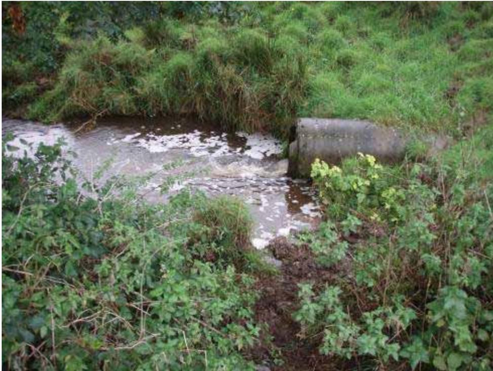
Photo 11 Culvert pipe on small tributary perched above downstream water level making upstream fish access difficult
