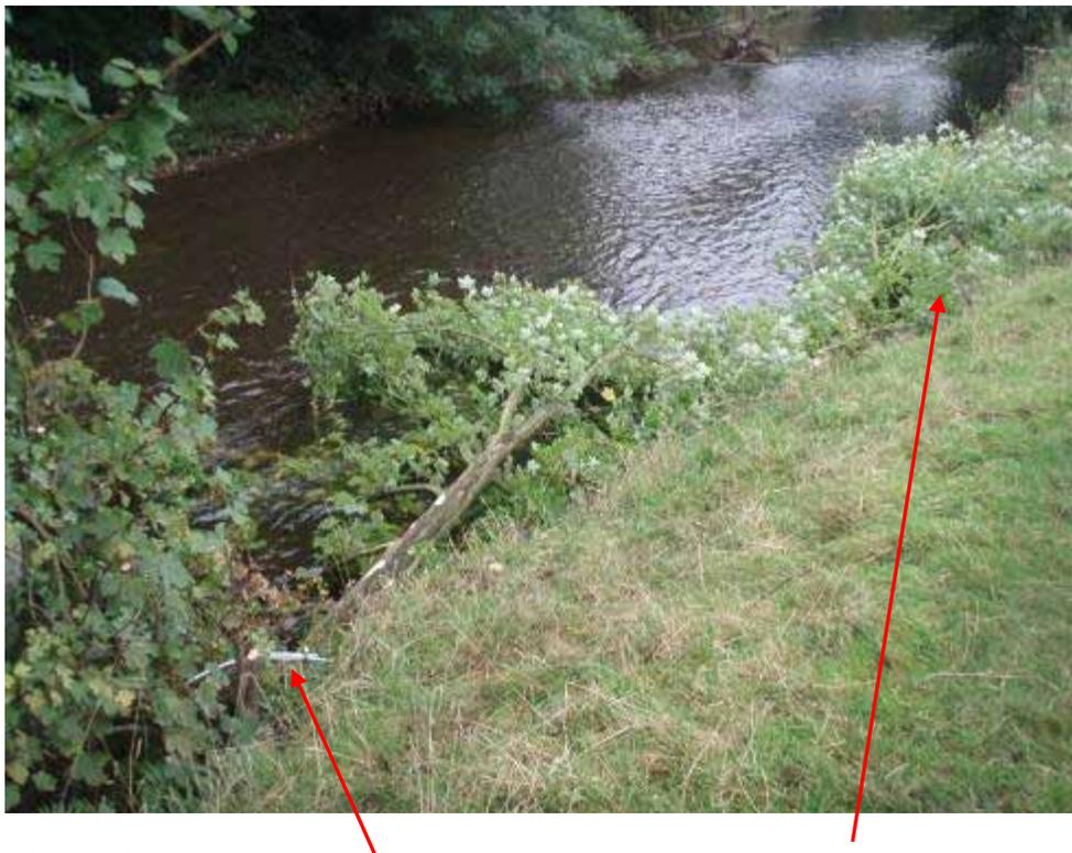
Photo 15 Tree kicker anchored to bankside tree with cable, protecting scalloped bank
