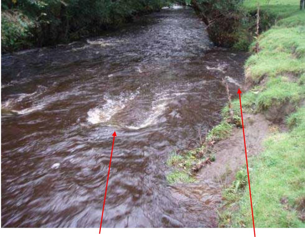
Photo 5 Boulder placed too close to right bank, causing bank erosion
