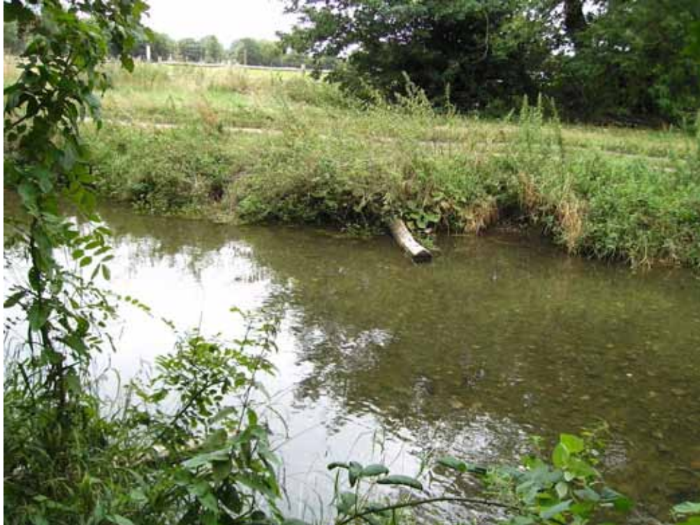
Photo 9: Previously installed upstream facing flow deflector (RHB) in Foots Cray Meadows. This particular structure is probably too small to noticeably influence flow heterogeneity and scour.
