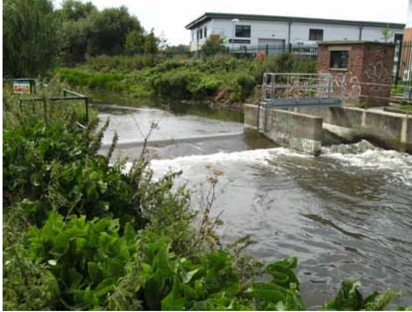
Photo 15: Weir at Crayford (in high flow conditions)
