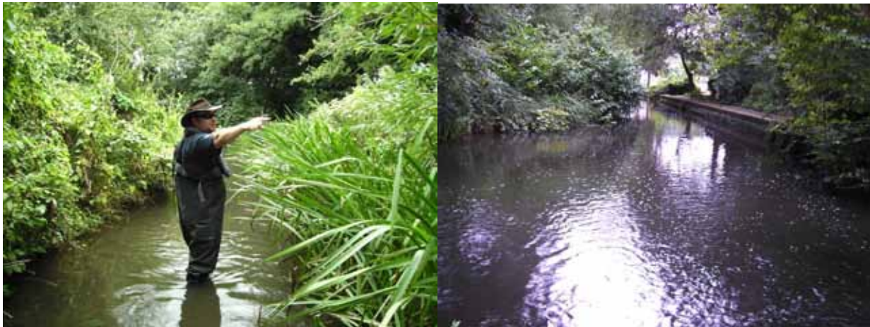
Photo 10: Narrower channel (left) and concrete modifications to channel (right)
